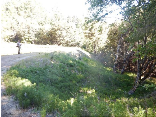
Photo 7: View of the pond berm and wetland vegetation
