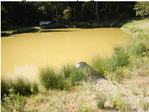
Photo 11: View of the pond outflow pipe looking towards the spring
