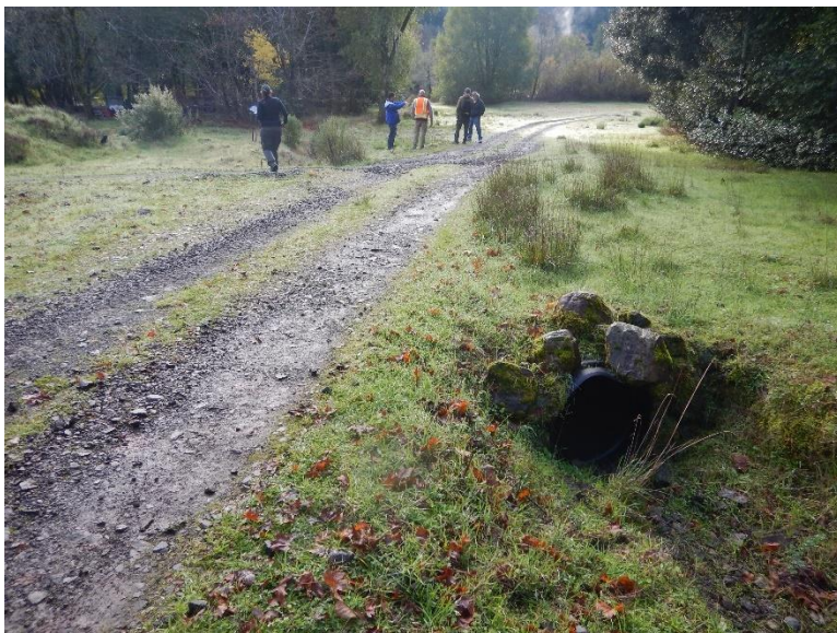
Photo 5, Crossing 6: Recently installed culvert stream crossing in low lying area
