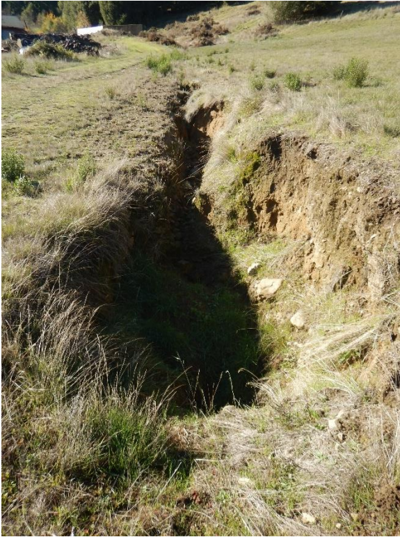
Photo 11, Culvert: Incising channel upstream of culvert crossing
