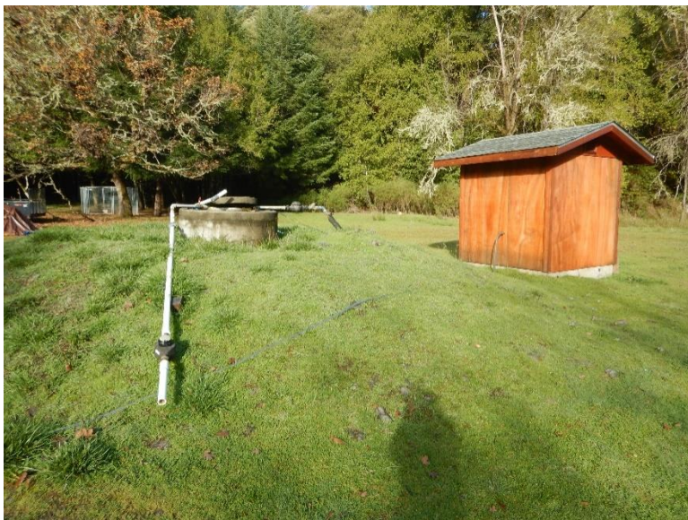
Photo 8, Well: Shallow well used for domestic and irrigation water
