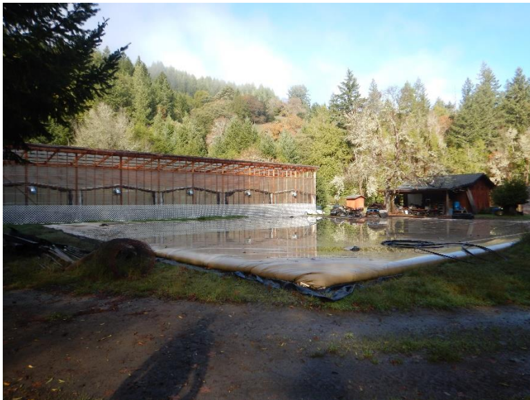
Photo 7, Water Bladder: Water storage bladder with no secondary containment system
