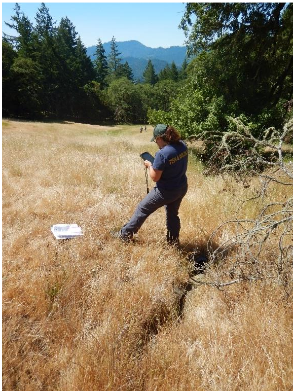
Photo 2: Wetland Culverts: Plastic culvert outlet in wetland area with entrenched channel downstream
