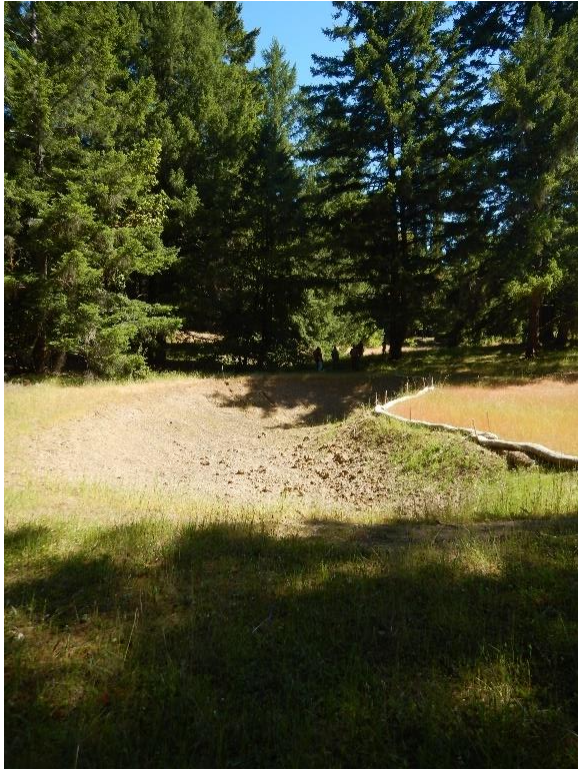
Photo 1: Pond: Partially constructed pond with staked straw wattles on downstream side
