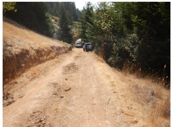
Figure 6. Road access to cultivation area concentrates stormwater downslope to the watercourse crossing.
