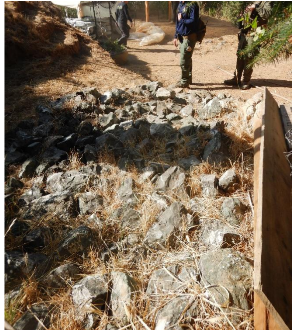
Figure 10. Rock placed in watercourse at WQ2.
