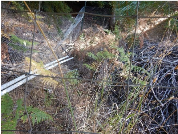
Figure 8. Debris on watercourse upstream of crossing at WQ2.
