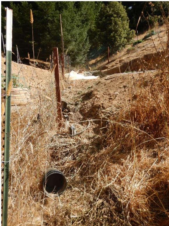
Figure 12. Culvert outlet at watercourse at WQ2.
