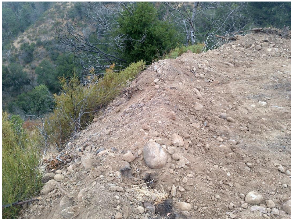
Photo 4—Earthen spoils at the edge of the road at WQ2.
