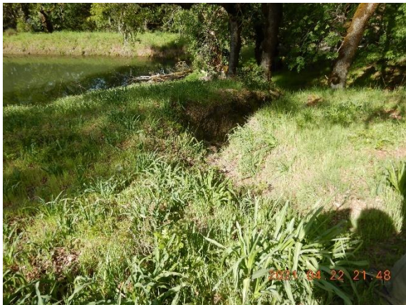
Figure 46. Scoured channel downstream of road and upstream of pond.
