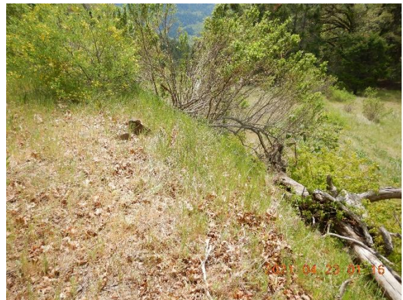
Figure 43. Fill slope of tank pad at 486 is steep.
