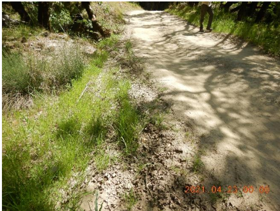
Figure 13. Drainage off road is directed to watercourse at WQ4.
