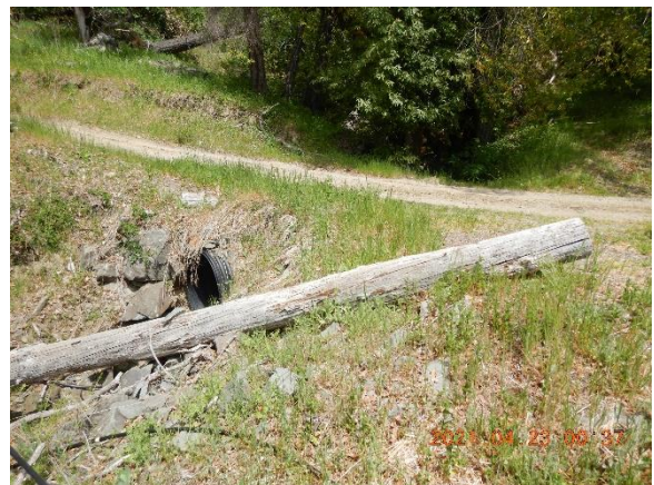
Figure 32. Class II watercourse crossing at 481.
