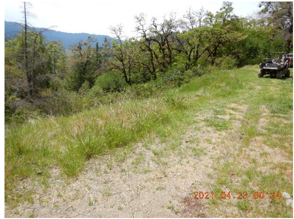
Figure 36. WQ8 – Fill slope looking north.
