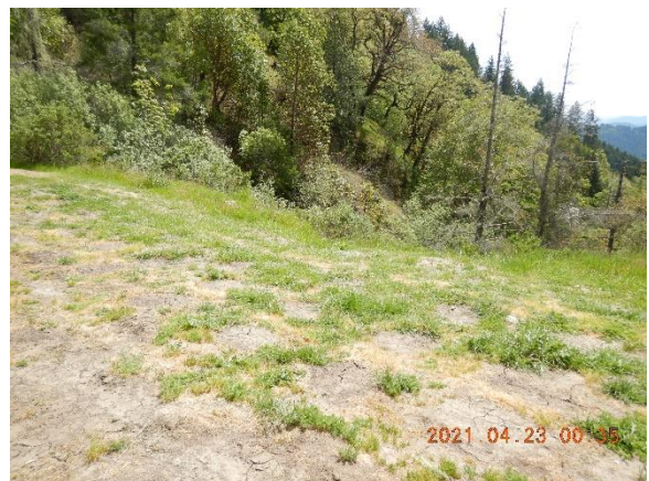
Figure 37. WQ8 – Fill slope looking west.
