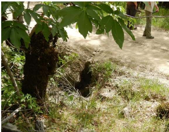
Figure 8. Culvert inlet with road surface connection.
