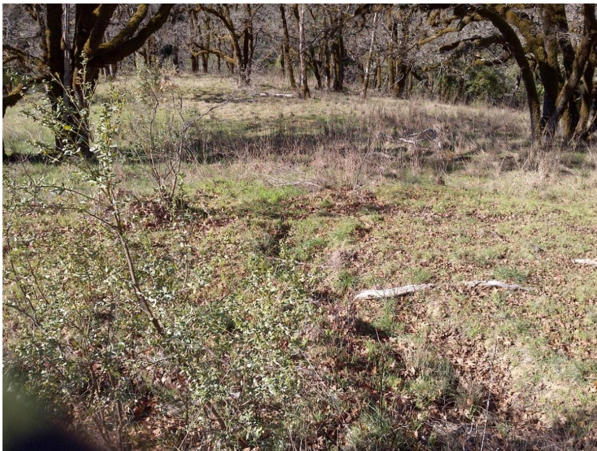
Photo 6—Looking southwest at the scoured channel from the southwest corner of the cultivation pad in the vicinity of RP 48.
