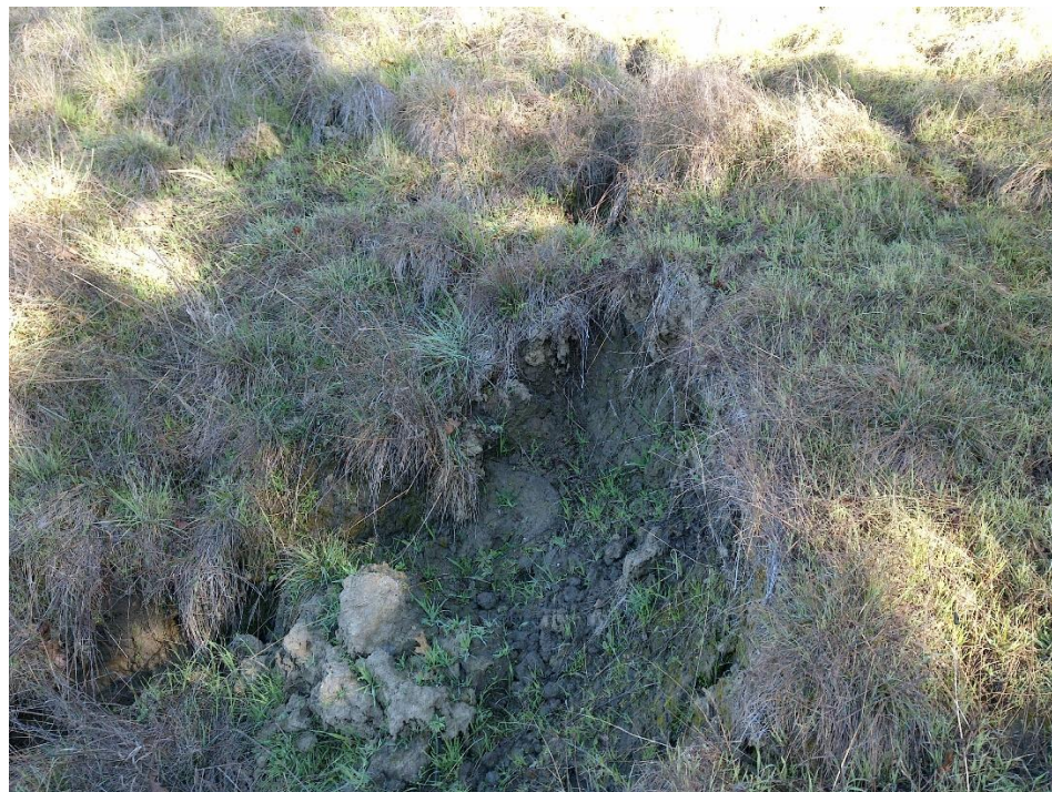
Photo 4—Looking upslope at a crack leading into a slumped block of soil. The crack continues to the clearly defined watercourse at the photographers back.
