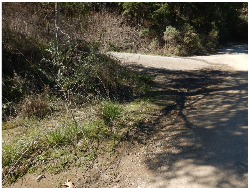
Photo 14—Looking west at the crossroads at RP 91. Water is present in the roadside channel despite no rain for more than a week.
