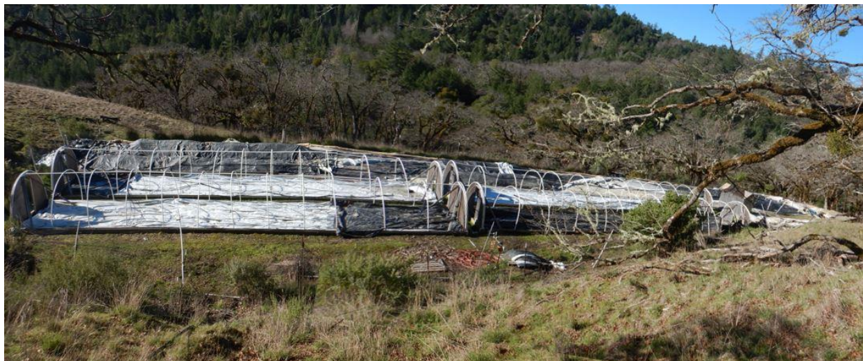
Photo 5—Looking southwest at the eastern side of the cultivation pad at RP 48.
