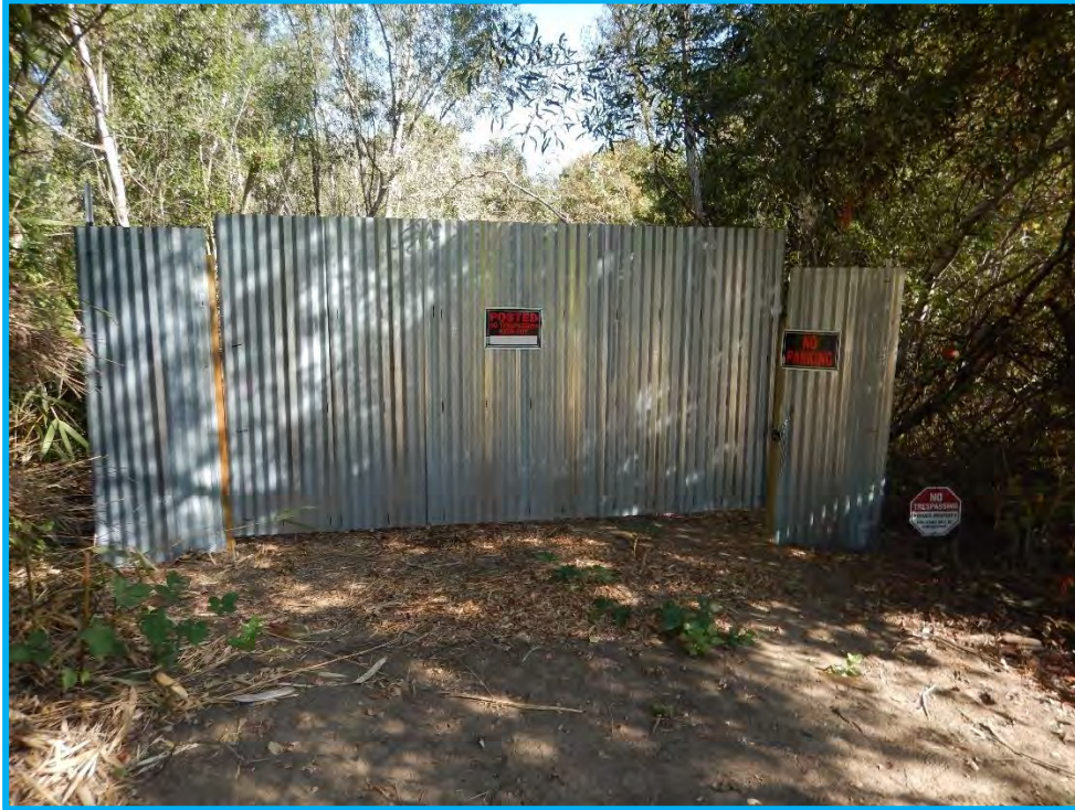
Photograph 1. New corrugated metal fence and gate installed at 9000 Mill Station Road, Sebastopol.
