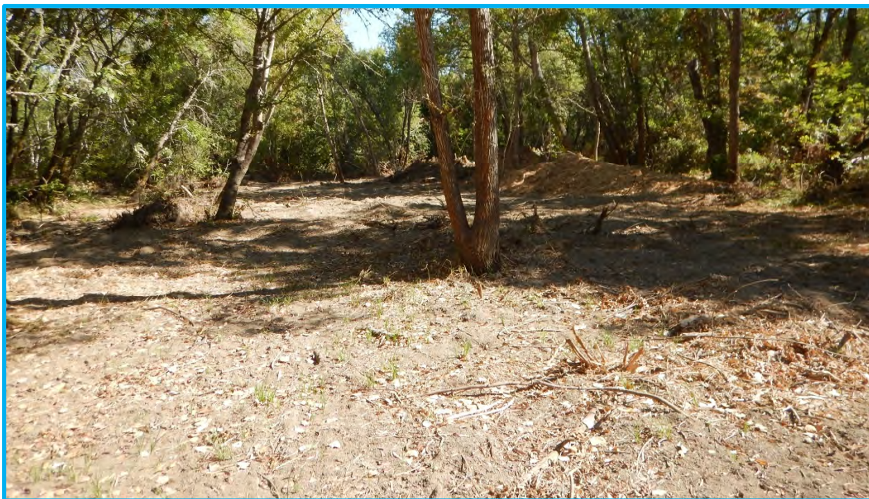
Photograph 13. Farther to the north, again, vegetation clearing was extensive, the soil surface was scrapped of all vegetation and the riparian trees were chipped with large piles of woodchips remaining on the eastern side of the clearing (right side of the photograph).
