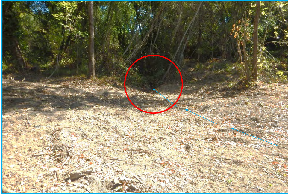
Photograph 19. Clearing and soil disturbance along the northern perimeter extended into a large overflow channel that significantly deepened and widened to the north. Sonoma County LIDAR Imagery shows the large overflow channel to merge with Atascadero Creek. The photo has been lightened to show the overflow channel and the channel circled in red. Blue arrows show flow direction during high water.
