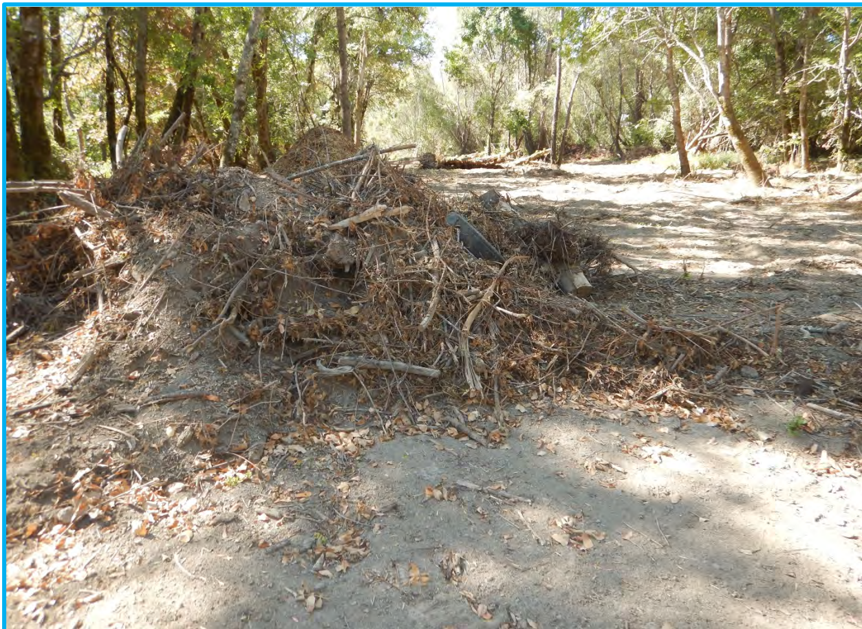
Photograph 15. Several large piles of scraped riparian vegetation and soil were left in piles along the eastern perimeter of the central clearing.
