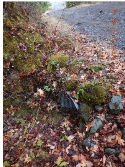
Figure 6. Class III watercourse crossing, culvert inlet at WP 607.
