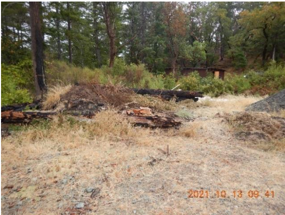
Figure 4. Edge of graded flat has debris and waste pushed over edge toward watercourse at WQ1.
