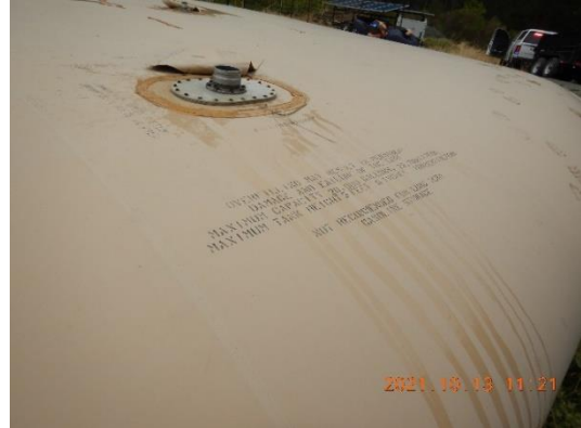
Figure 15. WQ2, Bladder without containment, with potential to runoff to and further erode Class watercourse at WQ1.
