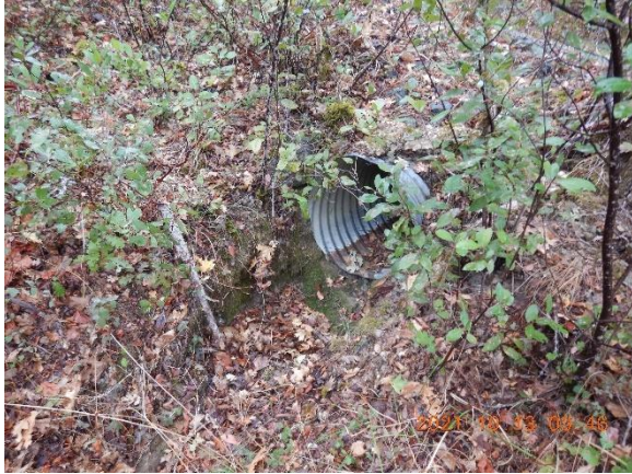
Figure 7. Class III watercourse crossing, culvert outlet at WP 607.
