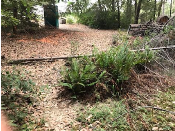
Figure 4. View of flowpath of sediment from access road to watercourse at WQ1. Watercourse runs left-right in photo, just upstream of the crossing. Note on the left, the porto-potty in the flowpath, and slash pile on watercourse, on right.
