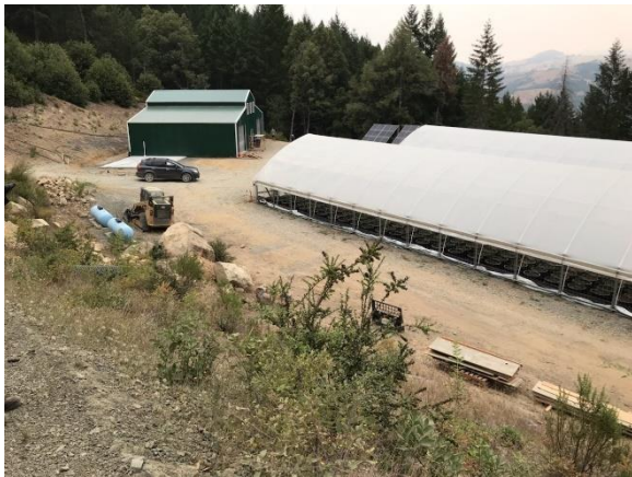
Figure 9. The inlet of DRC 2 is located on the outboard edge of the road, and the outlet discharges into the cultivation area.
