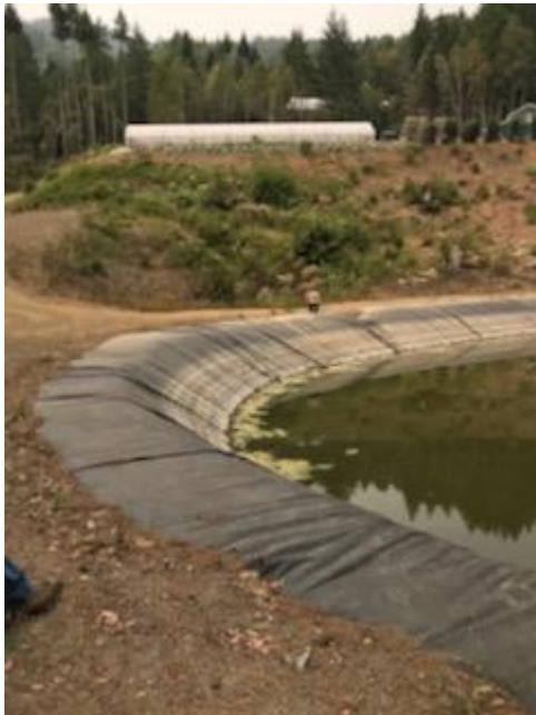
Figure 17. View of cut bank for pond flat. Road comes down on the left of photo, pond liner is in foreground. Spring is located at base of cutbank. Based on all descriptions and evidence, little earth was conducted to construct the flat, that the spring was already there, and known of prior to the pond construction.
