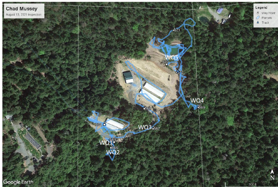
Figure 2. Inspection map for my August 13, 2021 inspection.
