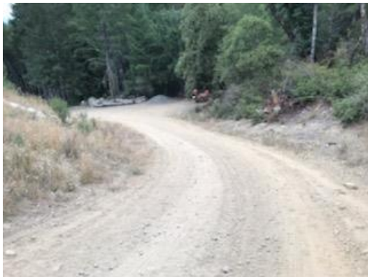
Figure 13. Steep road below second terrace, note pile of sand where stormwater can concentrate.
