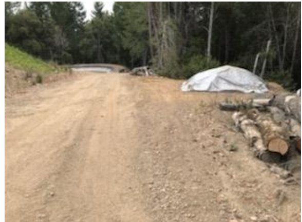
Figure 14. Steep road below third terrace to pond. Note soil pile where it can intercept stormwater runoff.
