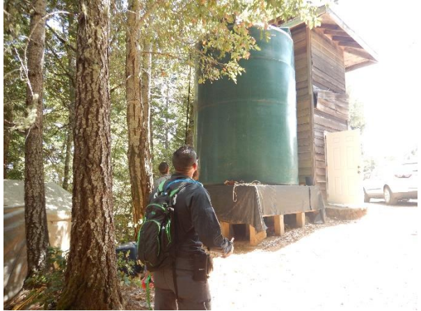
Photo 8: View of exterior water storage tank and tower with water tank inside.
