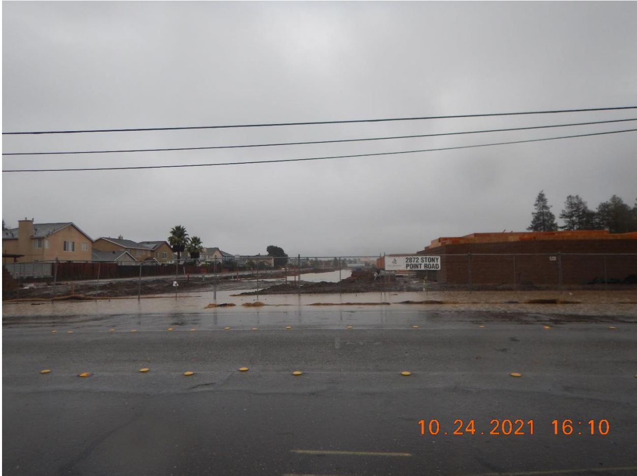
Photo 11: The North Entrance of the Project (Map 1), viewed from the west side of Stony Point Road. Turbid waters are emerging from the Site. There are no visible erosion controls on the earthen pads. Runoff is not effectively contained on the Site, and highly turbid waters are flowing from the Site beyond the installed wattles.
