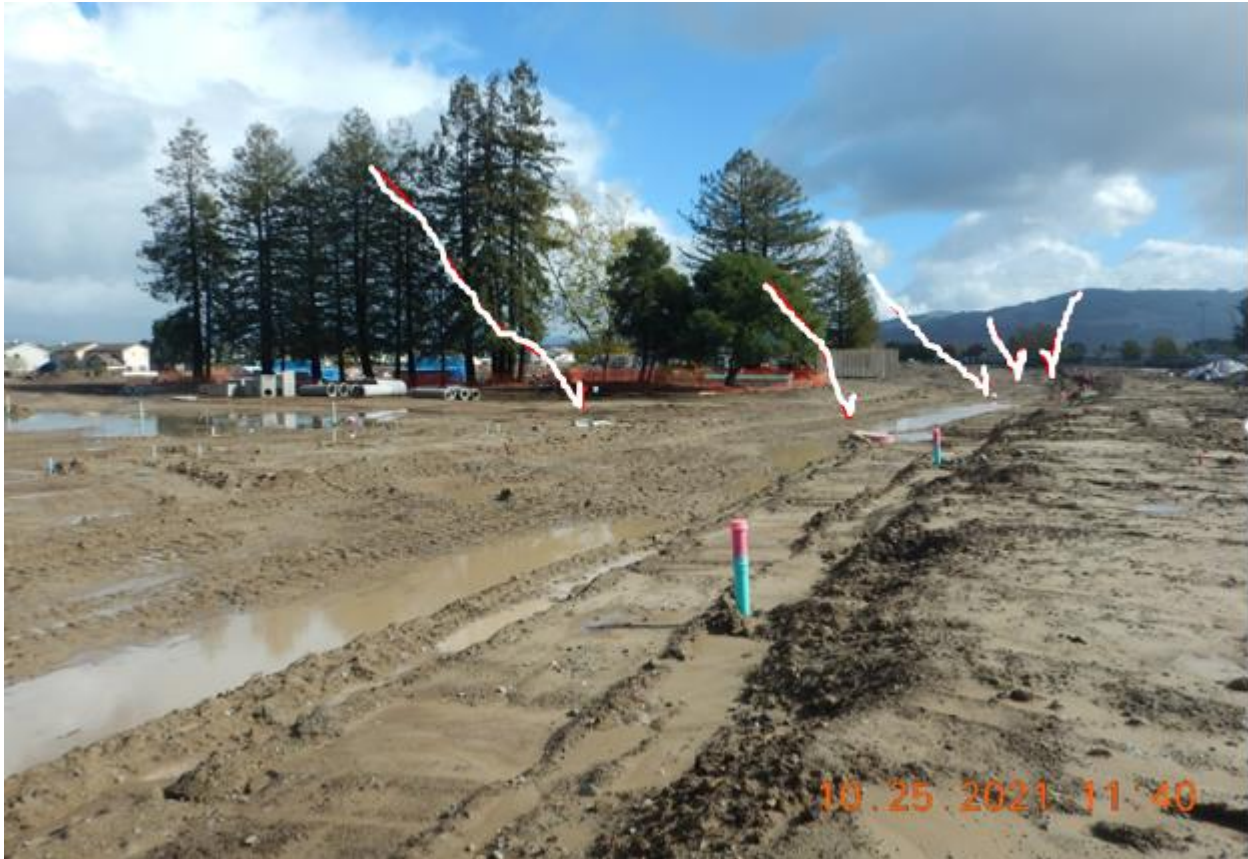
Photo 23: South side of Project area looking east-northeast. The road depression that was full of ponded turbid water the previous day (October 24, 2021) during the rain event is now almost empty. Not even the minimum erosion or sediment control BMPs are present on the Site. This entire area was under enough water the previous day that the manhole/storm drain inlet locations indicated with the white arrows were not visible.
