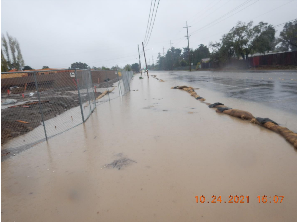
Photo 9: From Stony Point Road, highly turbid waters can be seen originating from the Site, consistent with my observations at the southern and northern mixing zones along Stony Point Road (Photo 5, Photo 6, Photo 7, and Photo 8).
