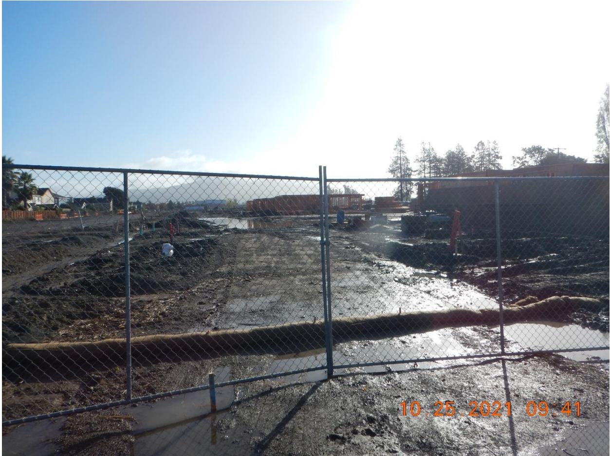
Photo 15: Looking into the Site from the North Entrance. Stormwater in the area where ponding stormwater was observed during yesterday's rain event has receded to a low spot near the center of the photo. The volume remaining in this photo is significantly less than what was observed yesterday, as seen in Photos 10 and 11.
