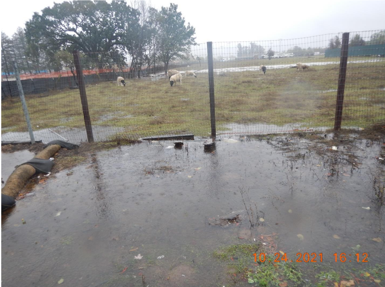
Photo 7: From Stony Point Road, I observed the adjoining property on the south side of the Project. Note the wattle in the foreground and the long black with orange fence that stretches the southern perimeter of the Project. Runoff from this neighboring property is low in turbidity. Note the clarity of the water: the leaves, grass, and the ground surface can be distinguished through the pooling stormwater.
