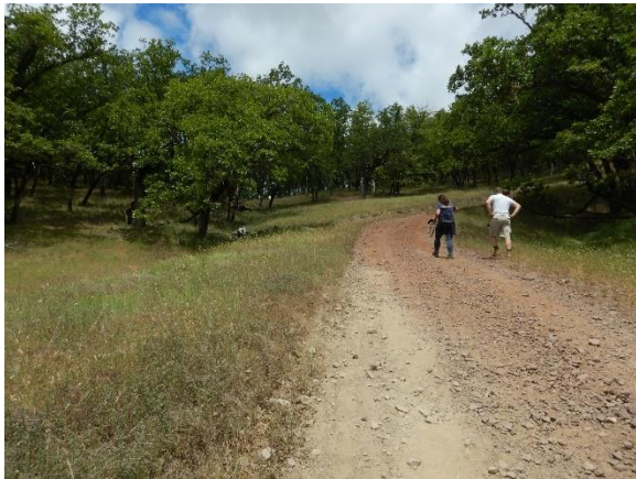
Photo 6: West Road: steep dirt road with no drainage structures
