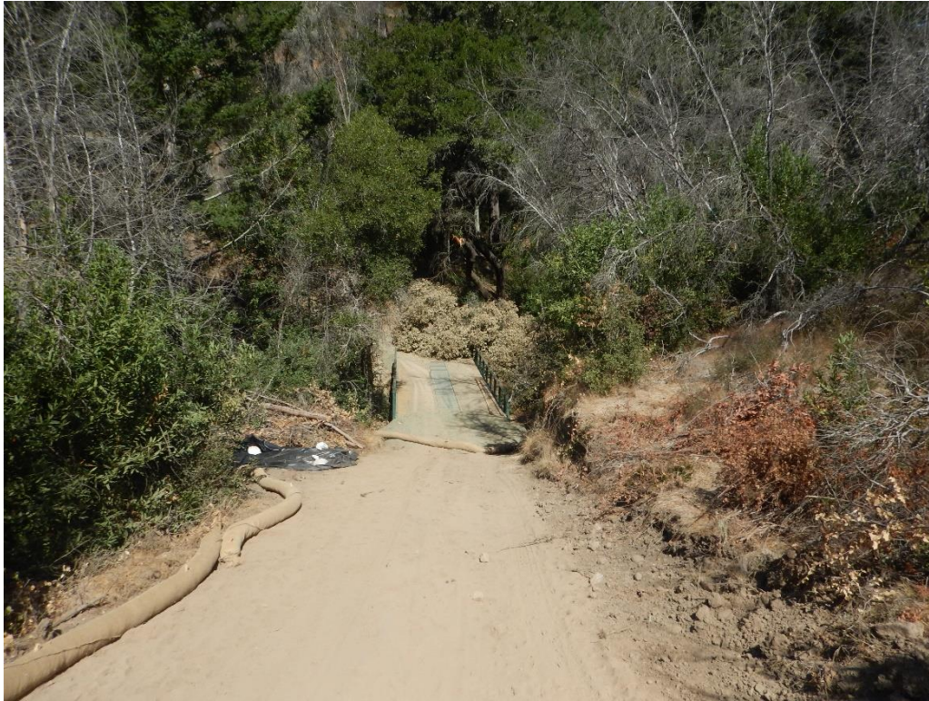
Photo 3. Recently installed bridge at WQ8 and opposite direction view of road and wattles in Photo 1.
