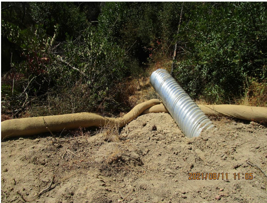
Photo 4. Outlet of recently installed culvert at WQ9.
