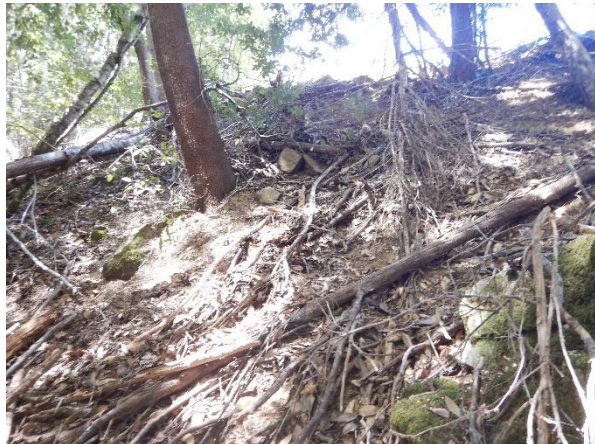
Photo 12: Closer view of CA2 graded area fill material above MP1.
