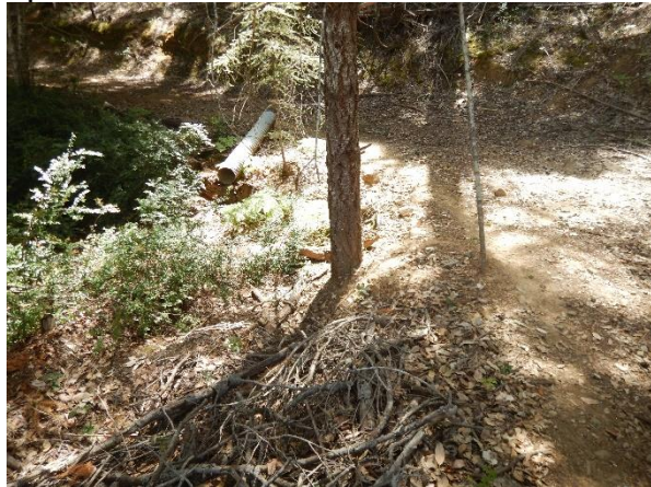
Photo 10: View of XNG2 outlet located upstream of MP2.
