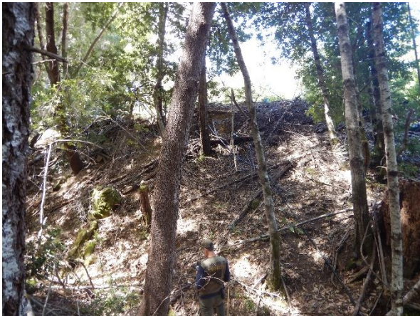
Photo 11: CA2 graded area fill material above the Class II watercourse and MP1.
