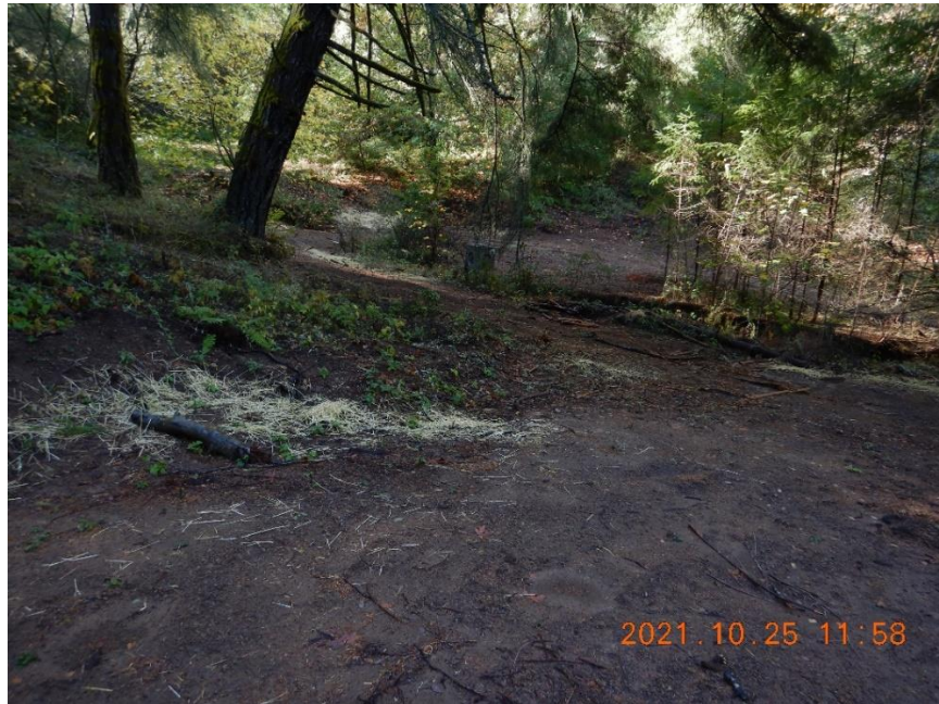
Photo 19—Looking west towards where a road crosses a watercourse at WQ12. A concrete cube (proposed drop culvert) is visible in the middle back of the image and a road can be seen passing between the concrete cube and a large tree.
