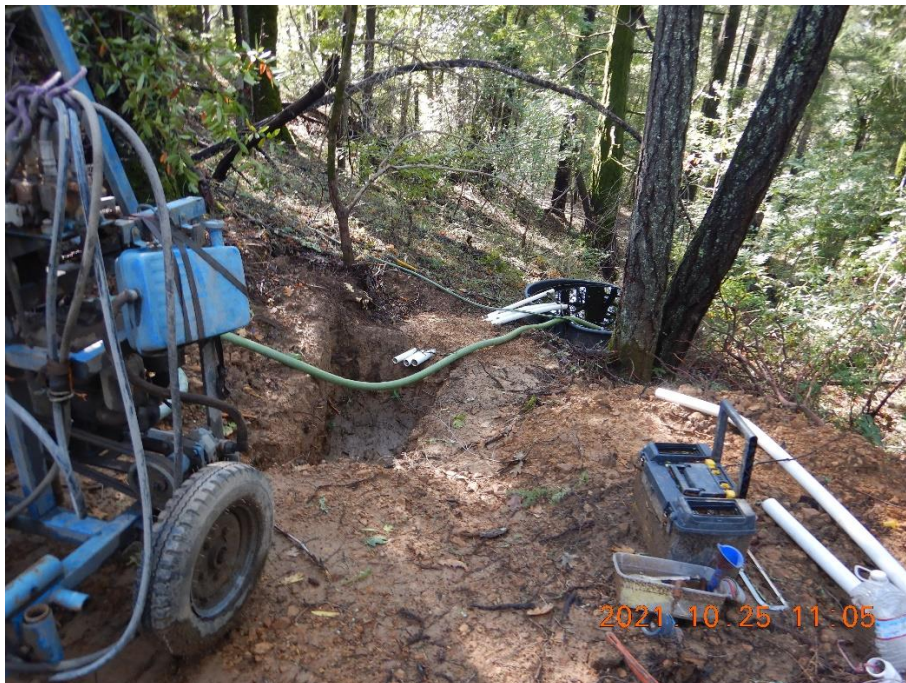
Photo 18—New well drilling location at WQ11. Mr. Vattuone advised staff that the drill core had broken off while drilling at the previous location and that the core was abandoned in the well.
