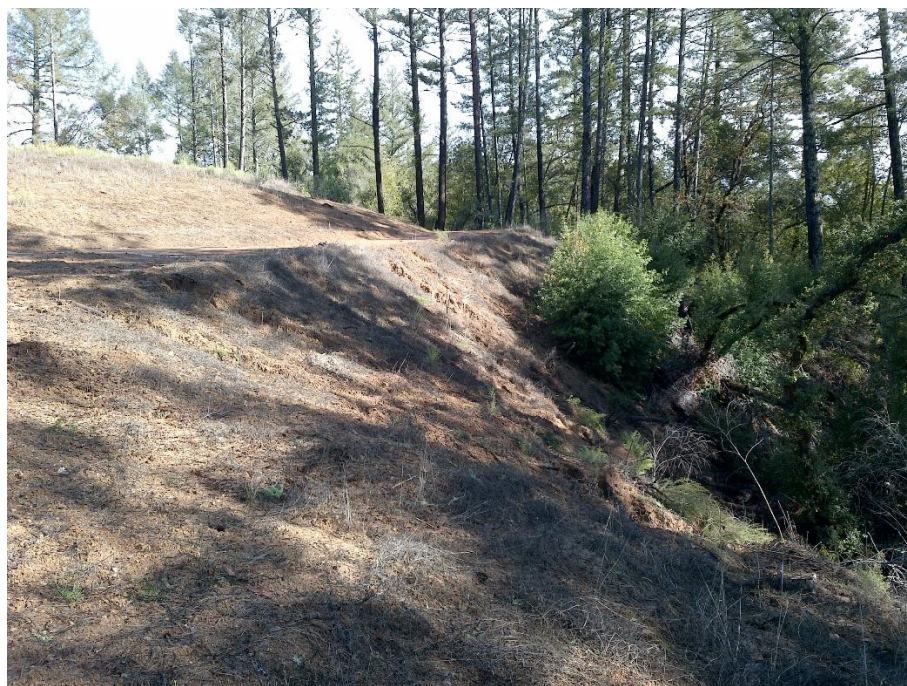
Photo 6—Looking north on the eastern edge of the pad in the vicinity of WQ5. Rills are visible on the east dipping slope in the middle of the image.
