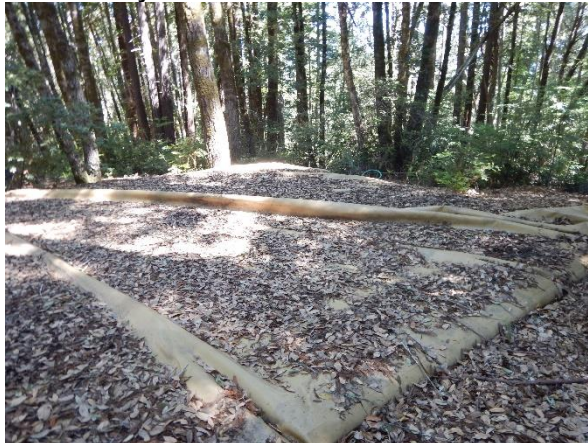
Photo 8: Water storage bladders without secondary containment.
