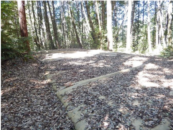
Photo 7: Half full water storage bladders without secondary containment
