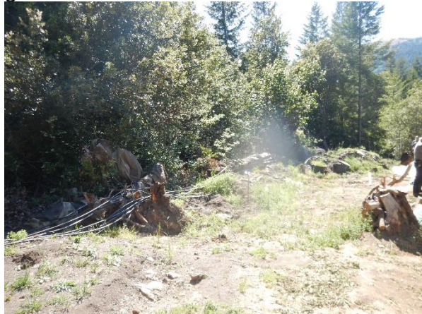
Photo 22: View of fill and slash the greenhouses.
