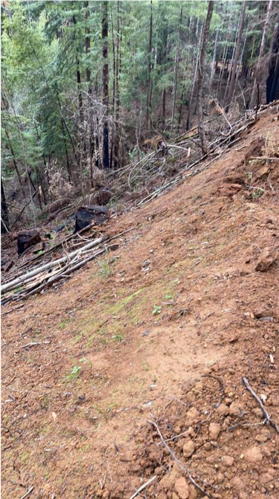
Figure 7. Sidecast material from newly removed waterbars near Water Quality Map Point 6.
