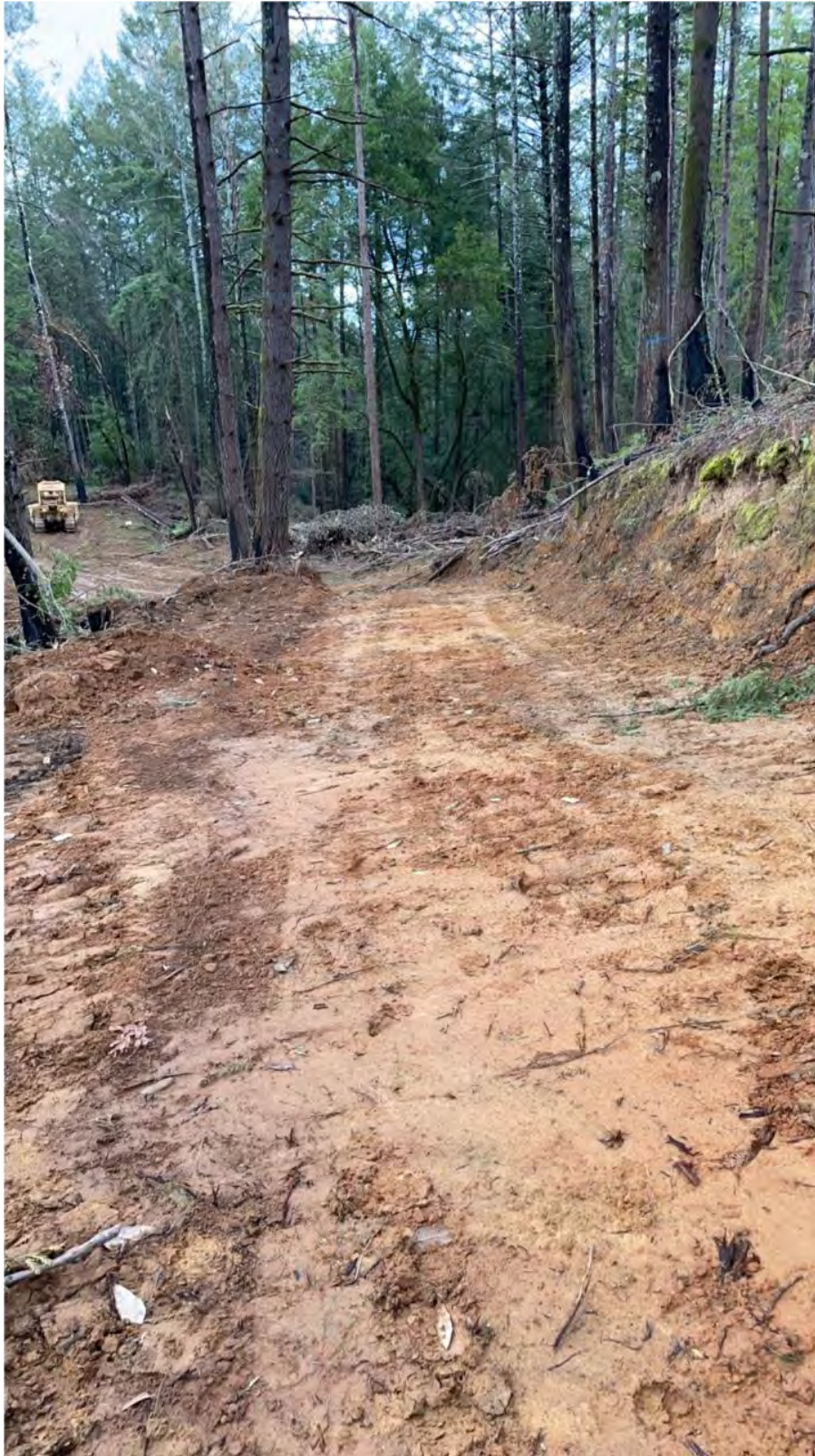
Figure 6. Newly Removed waterbars near Water Quality Map Point 6.
