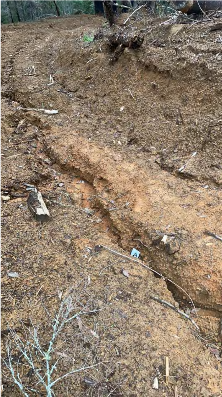
Figure 1. Road surface gulying at Water Quality Map Point 5.2. 6-inch Rite in the Rain card for scale.
