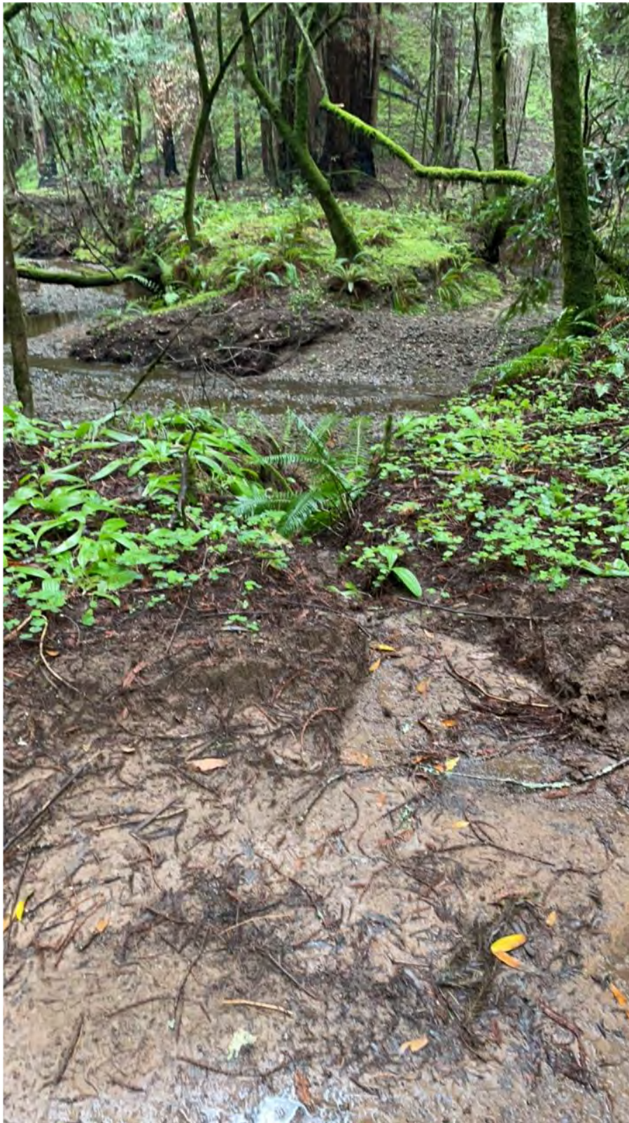
Figure 9. Class III diversion down road delivering to Felta Creek through breach in outboard fill near ICSP Map Point
