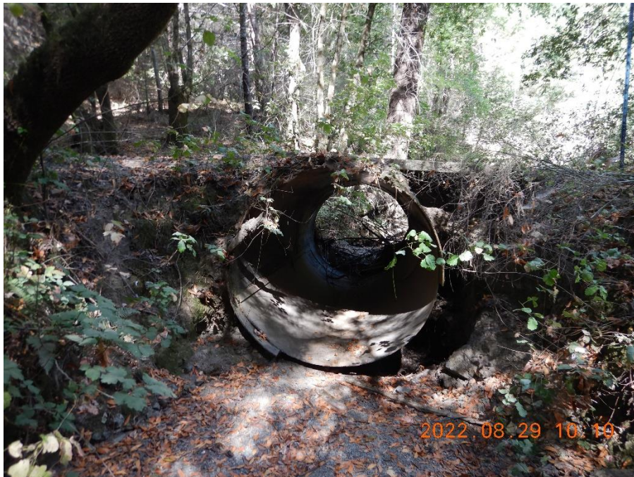
Photo 18—Looking north and upstream at the crossing pictured in the previous image. The culvert is six feet in diameter.
