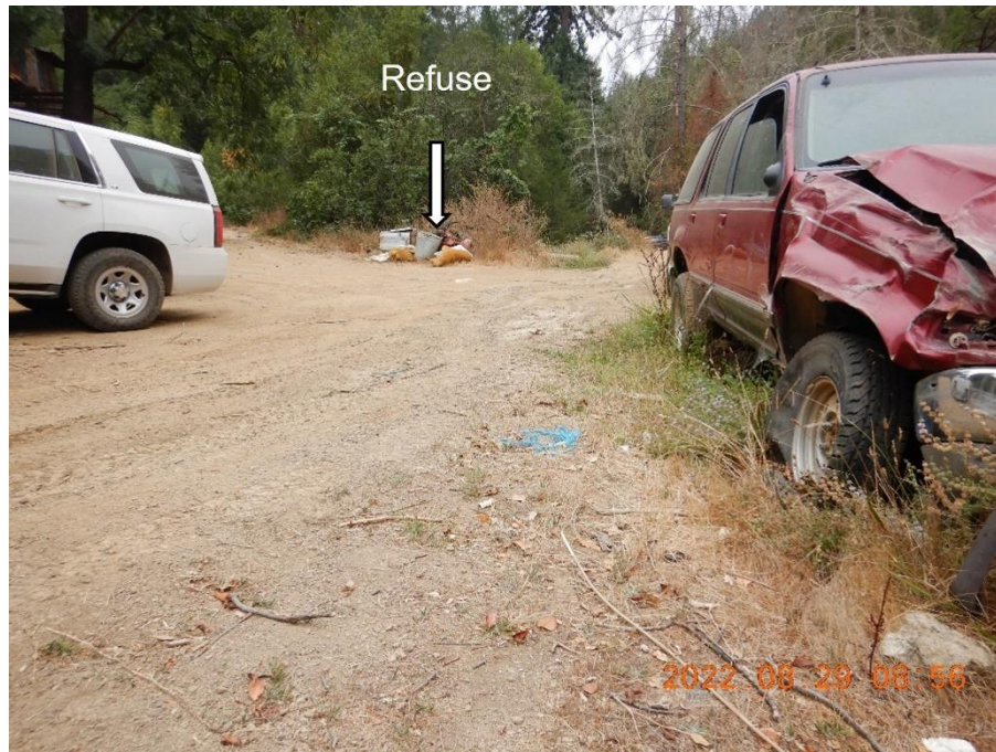
Photo 3—Looking south at WQ1. The tractor pictured in the previous image is to the back of the photographer. There is no culvert in this location and the topography is shaped such that stormwater will pass from behind the photographer to a receiving watercourse behind a pile of refuse in the top center of the image.
