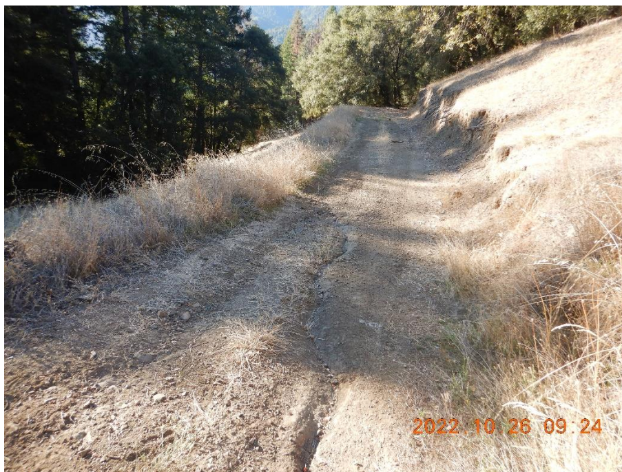
Figure 15—Looking south along the dirt road in the vicinity of WQ12. A sinuous scour mark is visible on the road's surface.
