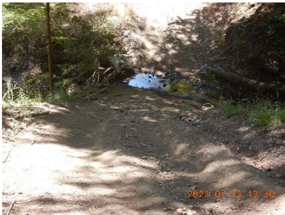
Figure 25. WQ5, WP803, Stream Crossing 2.
