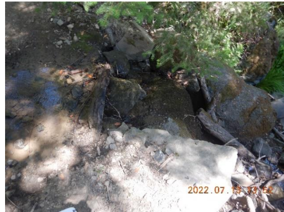
Figure 26. WQ5, WP803. The crossing consists of large rocks used to level the road surface, and a wet ford across the stream.
