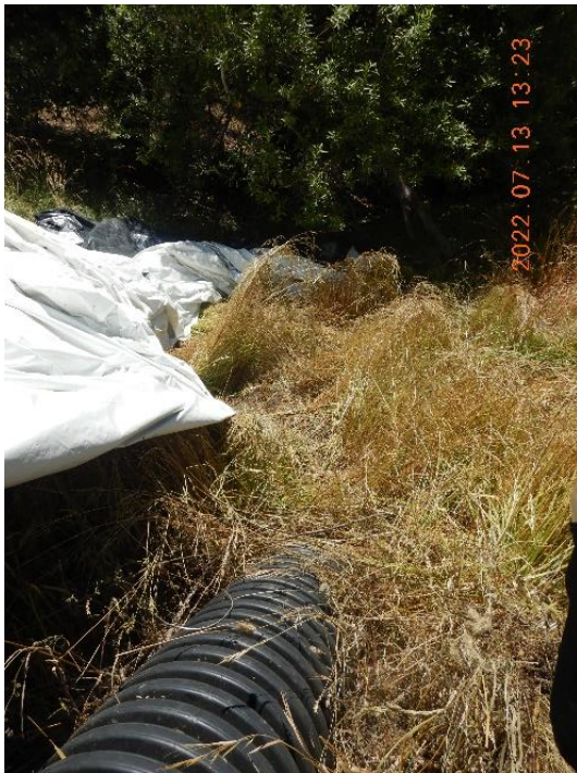
Figure 16. Outlet of culvert discharges onto fillslope of CA3 graded flat.
