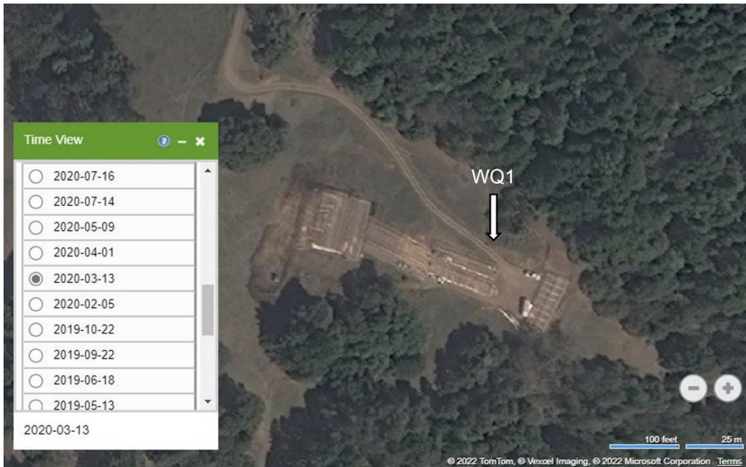
Figure 4 Aerial image taken on March 13, 2020, obtained from Land Vision services. Image shows greenhouses being constructed south of WQ1 where they impact a tributary to Tenmile Creek.
