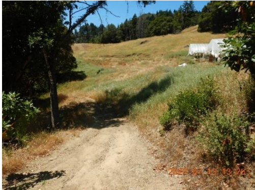
Figure 20. WQ3, WP 796. Road below CA3 with sediment delivery to a Class III channel.
