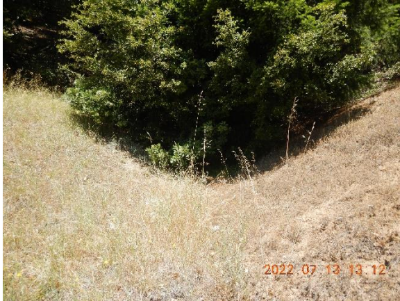
Figure 10. Swale above road at CA3, looking upslope.
