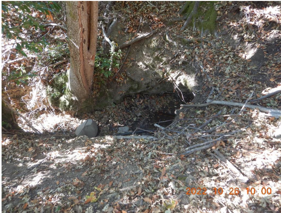
Figure 18—Watercourse located at WQ6. A black plastic pipe, visible in the channel, was diverting the surface water to a storage tank north of WQ7 to the east.
