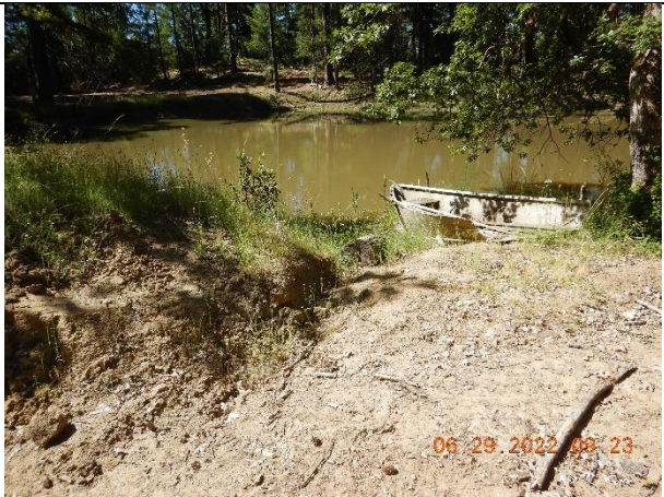
Photo 11: improperly designed overflow at inspection point WQ8
