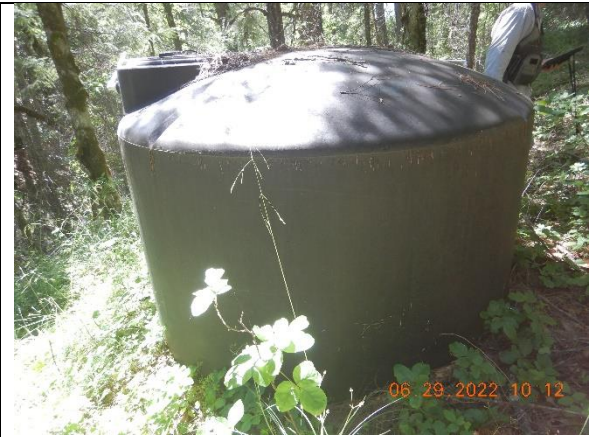
Photo 19: water storage tanks at inspection point WQ14
