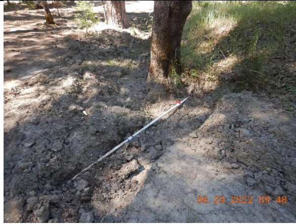
Photo 14: pipe out of the pond at inspection point WQ11
