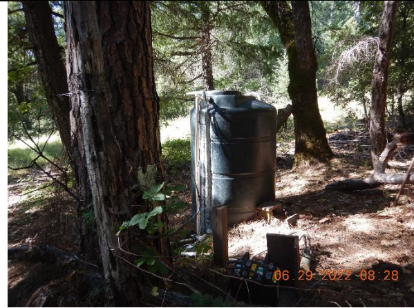
Photo 1: water storage tank at inspection point WQ1
