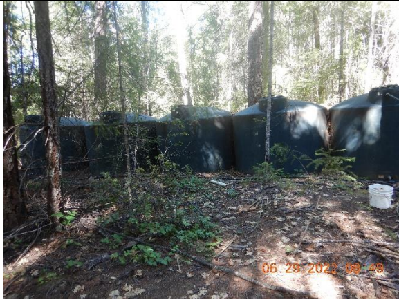
Photo 7: water storage tanks at inspection point WQ5
