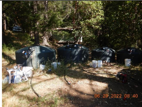
Photo 4: water storage tanks and a pump at inspection point WQ3
