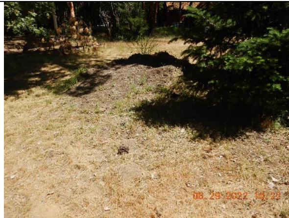
Photo 22: uncontained/uncovered soil nearby inspection point WQ17
