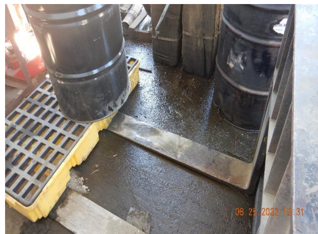
Photo 11a, 11b: Evidence of hydrocarbon spills within the roofed oil shed area. Picture taken by Farzad Kasmaei.
