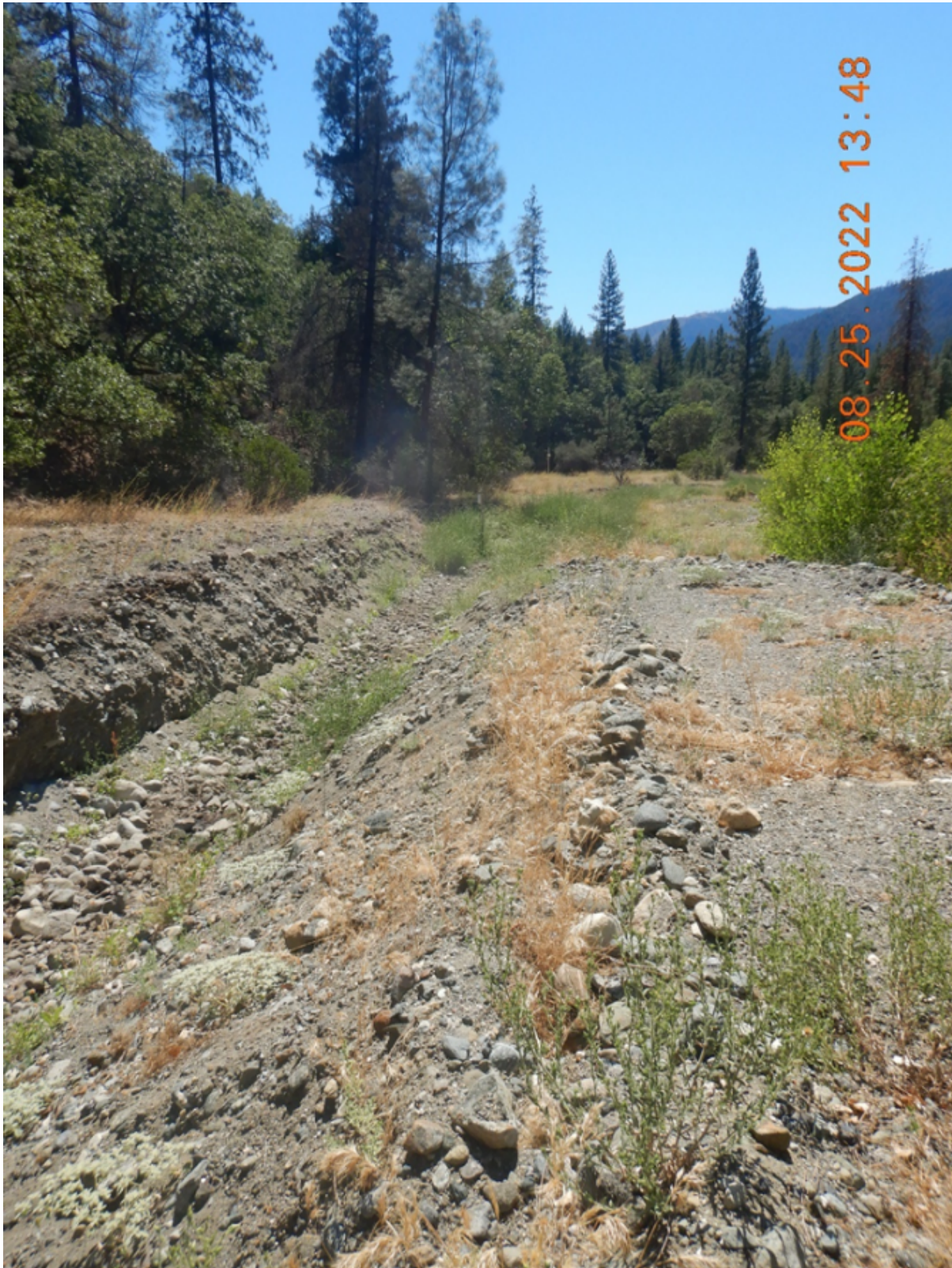
Photo 16a: channel modification in Oregon Gulch, facing downstream.
