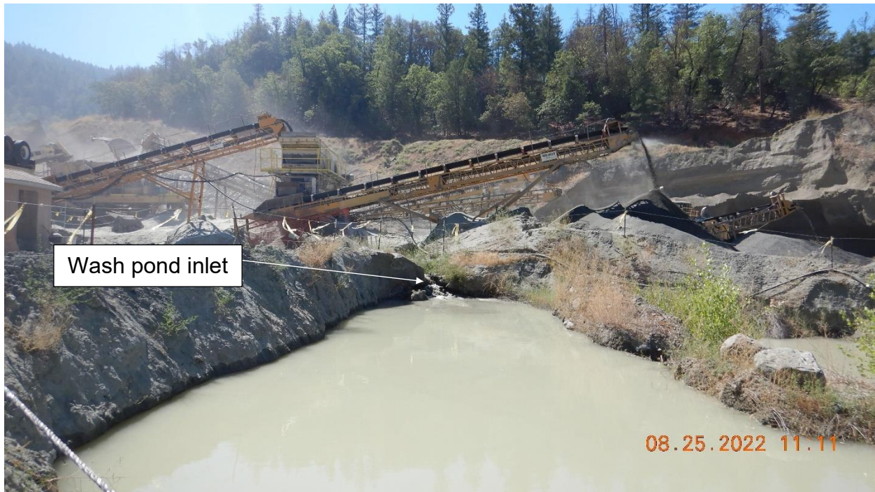
Photo 5: Looking south at the processing area where screening and crushing operations take place. The wash pond receives a highly turbid wash water from this area, and then it drains to a settling pond via a subsurface perforated pipe for further treatment. Picture taken by Farzad Kasmaei.
