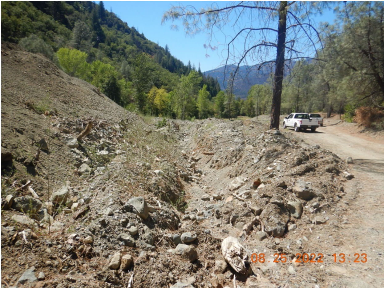
Photo 14a: Access road drainage crossing, facing downstream.
