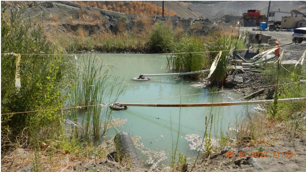
Photo 6: View of settling pond that receives wash water from the wash water pond via a perforated pipe. The water is mostly recirculated/reused. Picture taken by Farzad Kasmaei.
