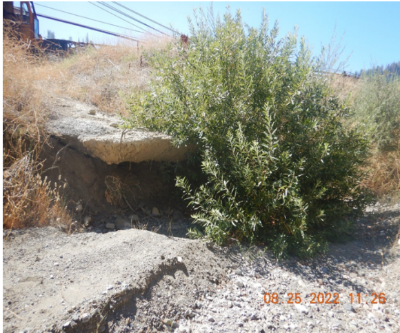
Photos 12a, 12b: Photo 12a concrete armor on left bank of Poison Gulch. Photo 12b concrete armor on right bank of Poison Gulch downstream of road crossing near office.
