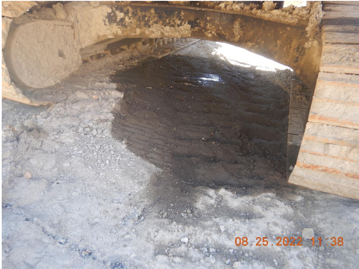
Photo 10: Evidence of hydrocarbon spills on the ground from a dozer near Poison Gulch. Picture taken by Amanda Piscitelli.
