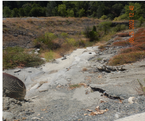
Photos 12a, 12b: Photo 12a concrete armor on left bank of Poison Gulch. Photo 12b concrete armor on right bank of Poison Gulch downstream of road crossing near office.
