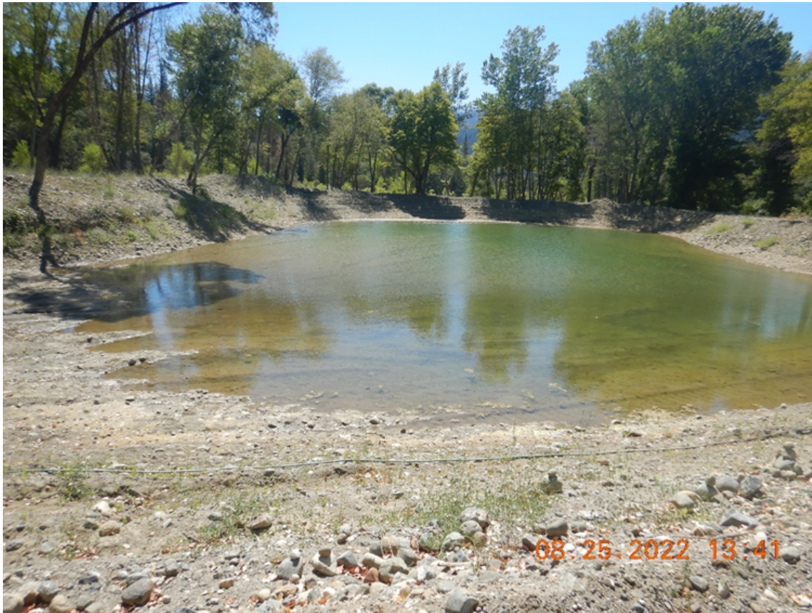
Photo 15a: Pond installed off channel, filled with water piped from Oregon Gulch.
