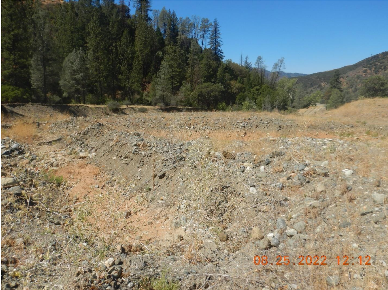
Photo 9: View of the installed wide berms in Oregon Gulch. Picture taken by Amanda Piscitelli.
