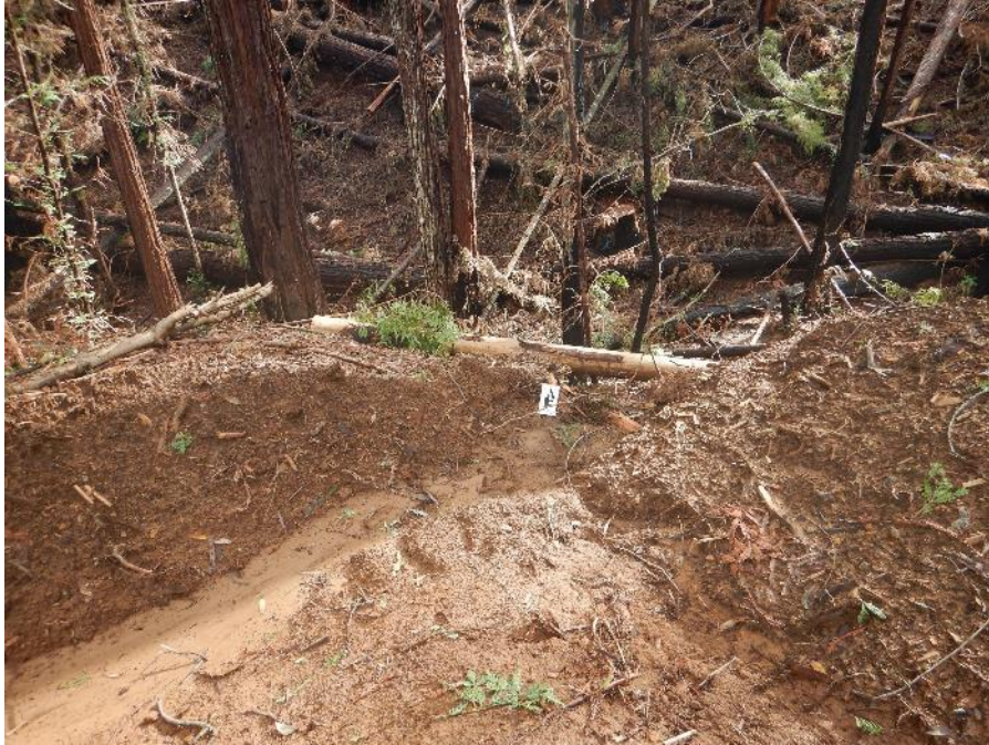
Photo Point 3.2 – Water and sediment reentering Class III watercourse after diverting down road and through sidecast material. 11/04/2021
