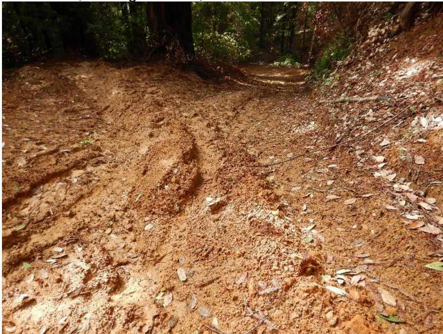
Photo Point 2.2 - Road, looking downhill, from first waterbar. 11/04/2021
