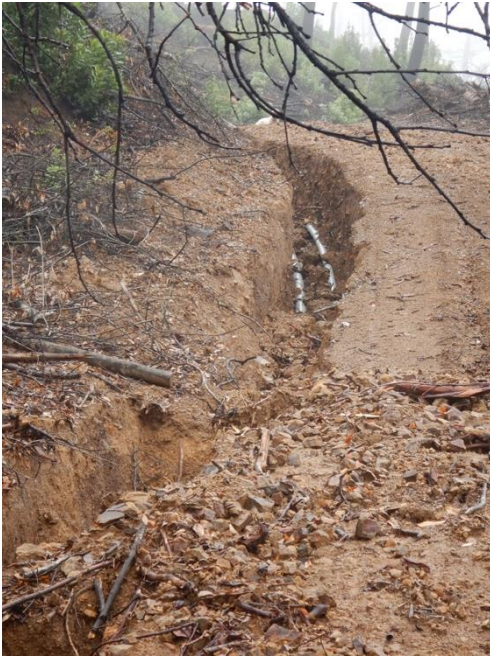
Photographs 1 and 2. The two photos show the washed out ditch line for the power cables. The ditch measures approximately 2 ft wide by 3 feet deep.
