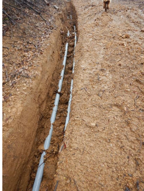
Photographs 1 and 2. The two photos show the washed out ditch line for the power cables. The ditch measures approximately 2 ft wide by 3 feet deep.
