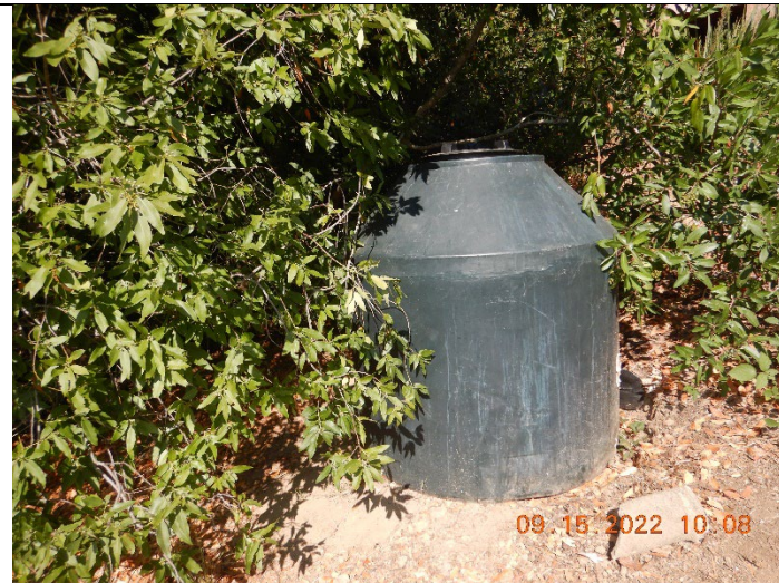
Photo 3: Water storage tank at inspection point WQ2
