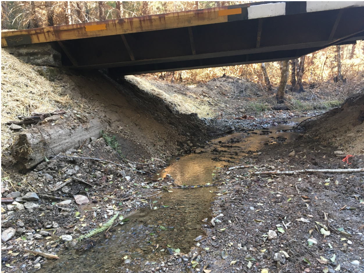
Figure 1: Looking upstream at the abutment on the north side of RP1.
