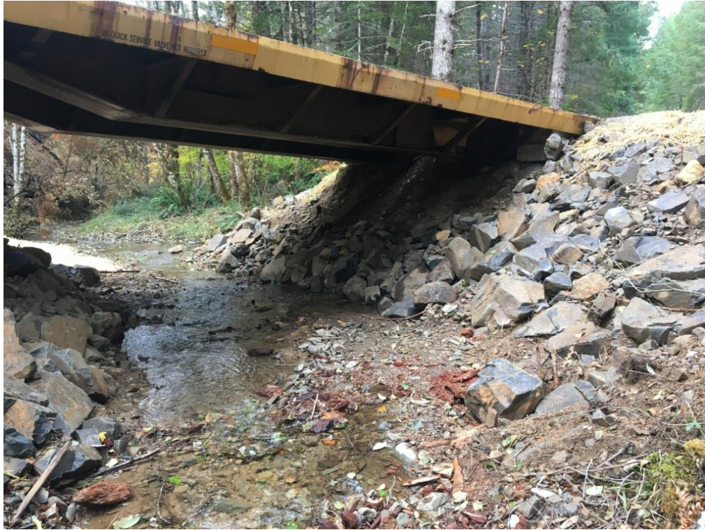
Figure 1. View of RP1 bridge from upstream facing downstream right bank.
