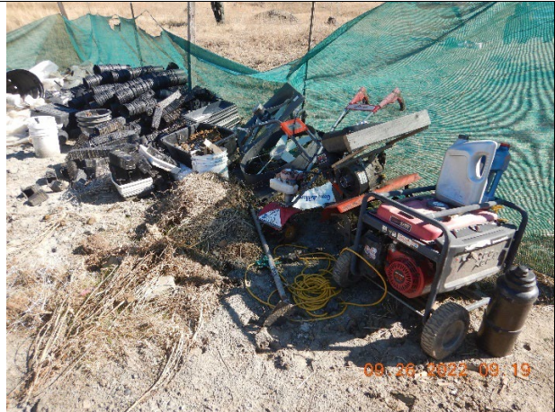
Photo 18 –uncontained generator and plastic containers in the vicinity of cultivation area at inspection point WQ2
