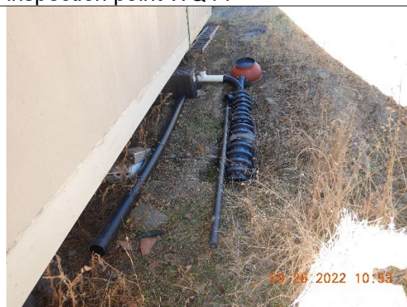
Photo 33 – Domestic wastewater pipe near a class III watercourse at inspection point WQ19
