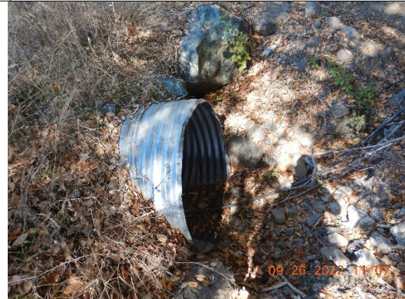
Photo 13 - A properly functioning culverted stream crossing at inspection point WQ26
