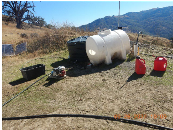
Photo 24 – Improperly stored gasoline tanks, water pump and water storage tanks at WQ9
