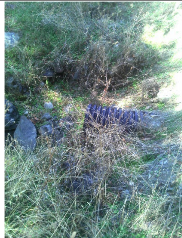
Photo 17 – Properly functioning culvert outlet at inspection point WQ31
