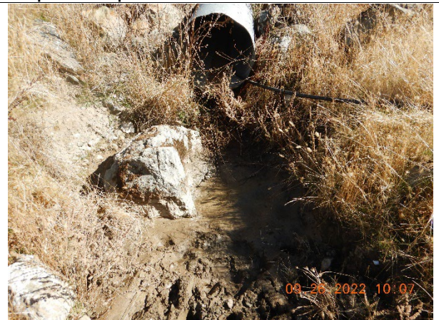
Photo 10 - Culvert outlet showing sediment delivery at the stream channel at inspection point WQ8
