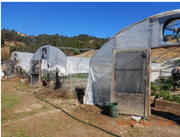
Photo 3 – Cannabis cultivation greenhouses within the required setback of a watercourse at inspection point WQ12
