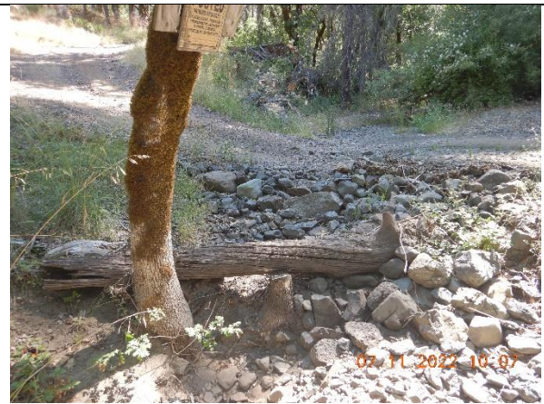
Photo 5: A rocked ford crossing at inspection point WQ6
