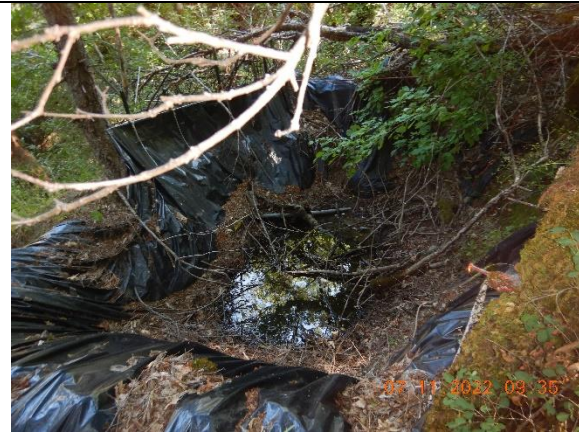
Photo 3: Impoundment at inspection point WQ3
