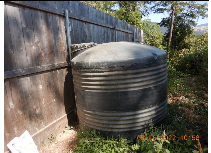
Photo 2: Water storage tank at inspection point WQ1
