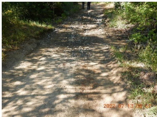
Figure 19. WQ4, WP771, watercourse crossing X3. The ford is 22' long by 8' wide.
