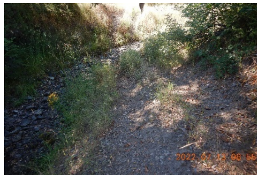
Figure 23. WQ5, WP772, watercourse crossing X4. The road approaches are hydrologically connected to the watercourse.
