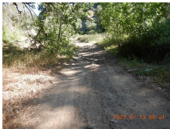
Figure 18. WQ4, WP771, watercourse crossing X3 is a ford crossing on Grub Creek. The unsurfaced road approaches are hydrologically connected to the watercourse. Outside of the crossings, Grub Creek is a free flowing stream.
