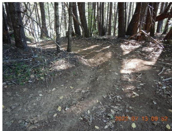
Figure 52. A road up to water tanks is very steep (30-50% slope) with wheel track troughs.
