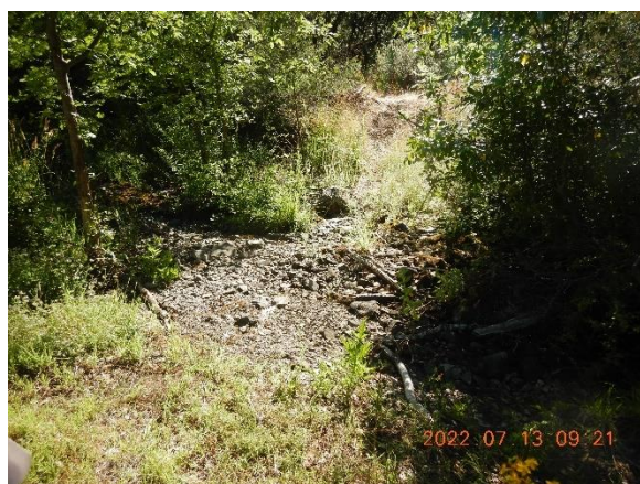
Figure 49. WQ11, WP778, quad trail watercourse crossing X5 over the Class II unnamed tributary. The ford is 12' wide by 6' long and connects to the crossing identified at WQ5, WP772.
