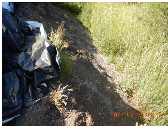
Figure 34. Pushed fill and potting soil encroaching over slope into wetland feature. Looking approximately south.
