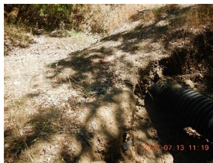
Figure 73. WQ17, WP 787. Misaligned corrugated plastic pipe located on a skid trail with eroded fill on tributary to Grub Creek
