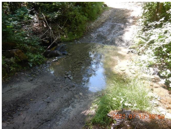
Figure 70. WQ14, WP 784. Ford crossing of Cold Creek. Both road approaches discharge to this stream this stream, shown as a blueline stream on the USGS map in Figure 3. 12' long wet ford built up with rocks in the channel. Lots of fine sediment deposited in channel.
