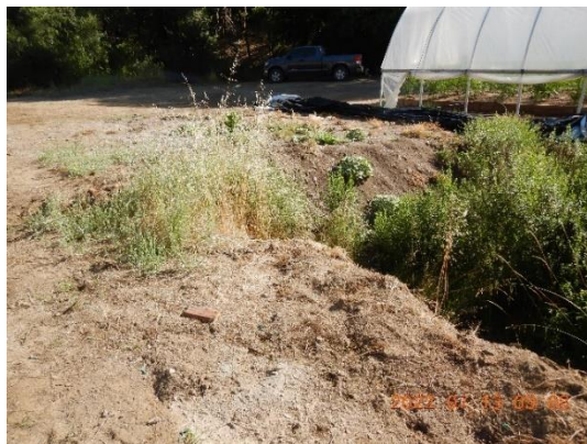
Figure 32. WQ8, WP776. Pushed fill encroaching over slope into wetland feature. Looking approximately north.
