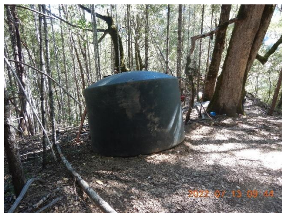
Figure 57. WP780. Water tank is not level.
