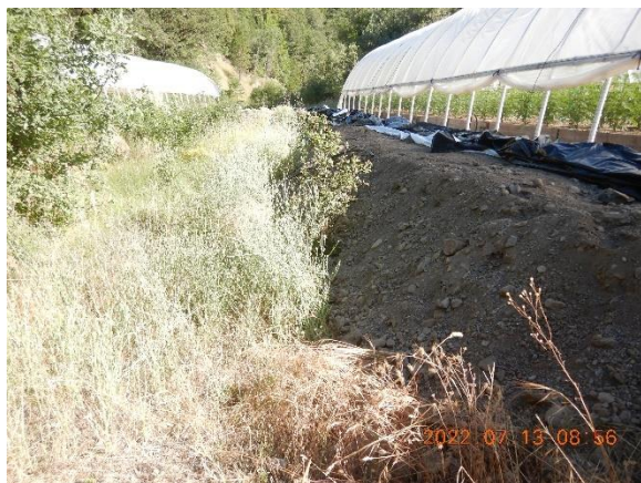
Figure 30. WQ8, WP776. Loose fill associated with the greenhouse pad construction is pushed over the break in slope with the wetland. Looking approximately north.
