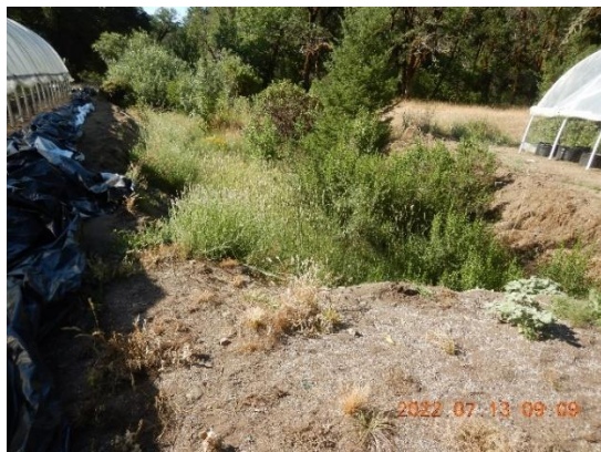
Figure 33. WQ8, WP776. Pushed fill encroaching over slope into wetland feature. Looking approximately south.
