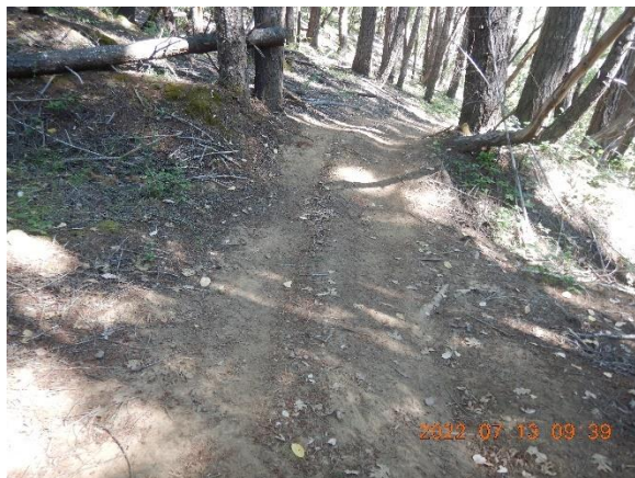
Figure 53. Road surface erosion has transported into swale at WP779 along road to water tanks.
