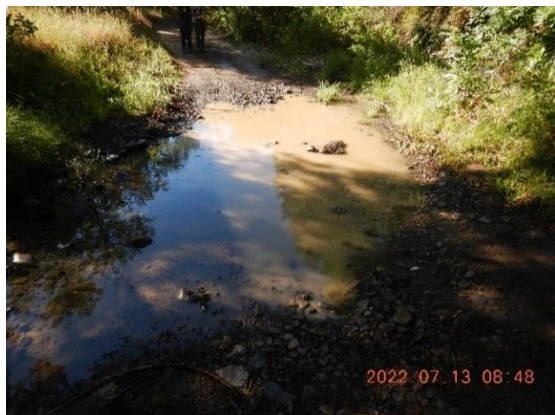
Figure 15. WQ3, WP770, watercourse crossing X2. Ford crossing on Grub Creek. 22' long by 12' wide. Vehicular use of the crossing results in a visible turbid plume downstream.
