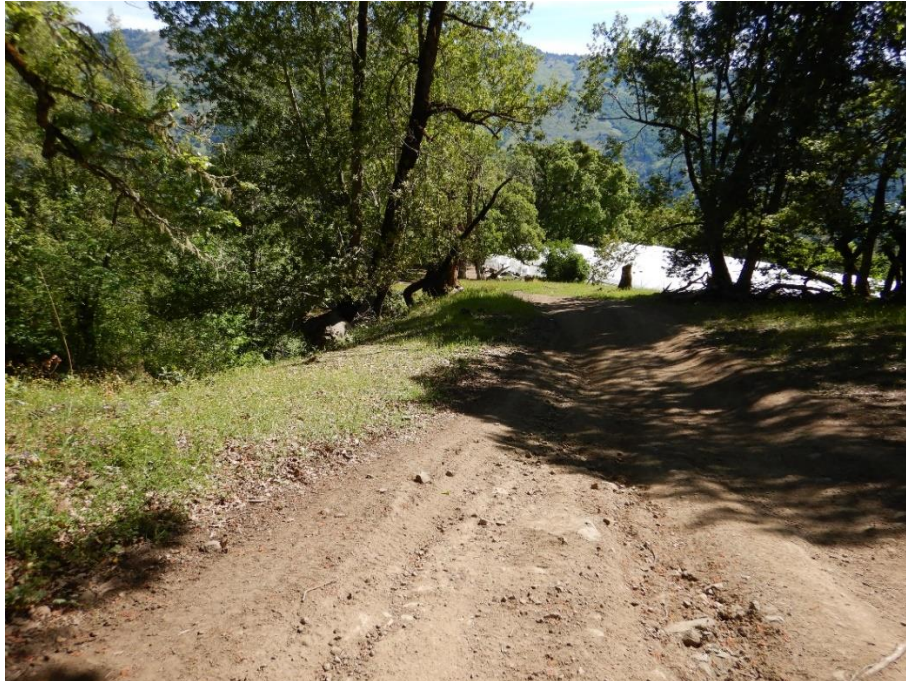
Photo 21— Looking east along road leading to WQ6. Road ruts connect to rills exiting the road in the middle back of the image, enabling stormwater to transport road pollution to a watercourse to the left of the image.
