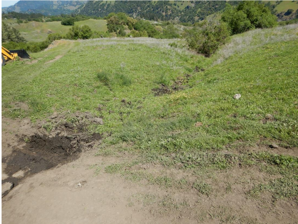
Photo 29—Looking north where saturated ground pictured in previous image connects to a watercourse tributary to the Eel River.
