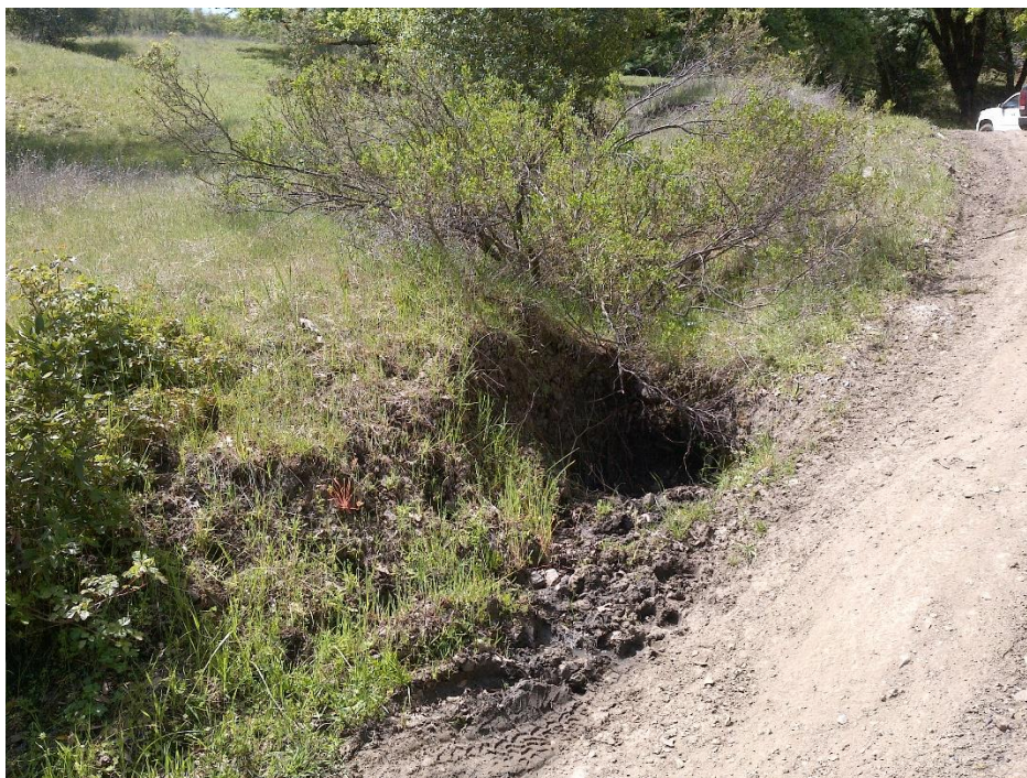
Photo 45—Looking upstream from road fording watercourse between WQ8 and WQ11.
