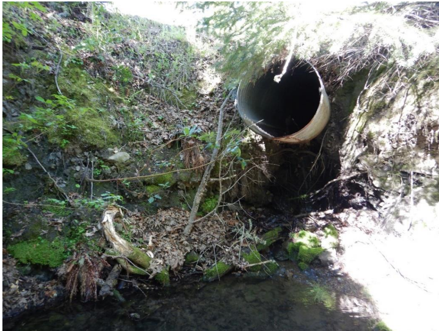
Photo 9— Looking upstream at outlet of culvert pictured in previous image at WQ3. The culvert outlet is perched 5 feet above the stream bed and has rusted through the bottom.
