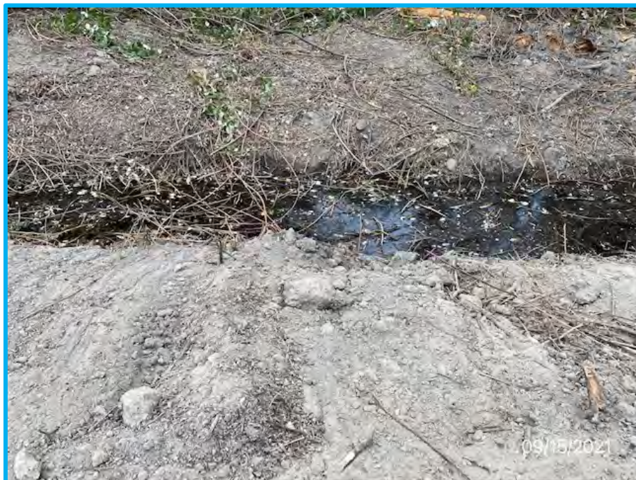
Photograph 4. Taken September 15, 2021 by Jackie Crawford showing Canfield Creek cleared of vegetation, earthwork within the wetted channel, and remaining Himalayan blackberry vines.
