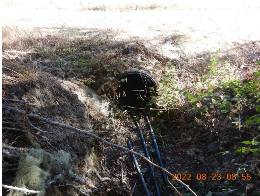
Photo 6— Looking north at the culvert inlet located at WQ3
