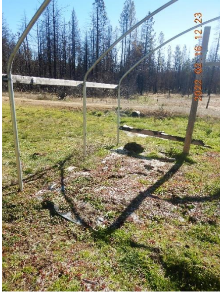
Figure 7. View from within greenhouse frame of access road running along southern Property boundary and inlet of Culvert 2. Vegetation, location, and hydrology suggest potential associated wetland areas.
