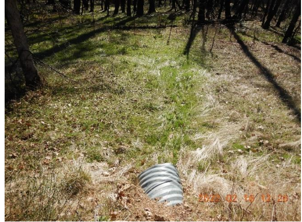
Figure 9. Culvert 1 outlet.
