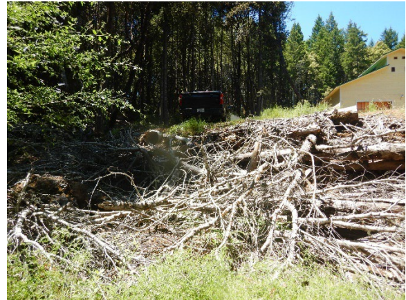
Figure 28. View of outlet of corrugated metal pipe and slash at the outboard edge of the landing.
