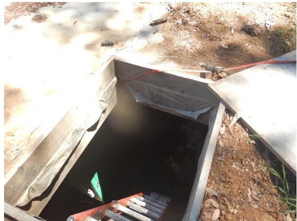
Figure 22. Buried shipping container is accessed from above via trap door.
