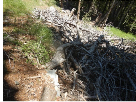
Figure 27. View of outlet of corrugated metal pipe, which extends from within the buried shipping container to the outboard edge of the landing.
