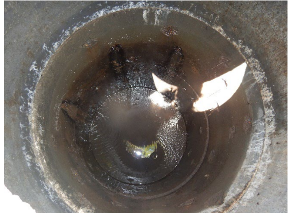
Figure 47. Interior of cistern at point of diversion.
