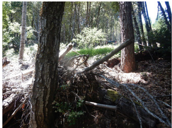
Figure 34. Steep slope below fill.
