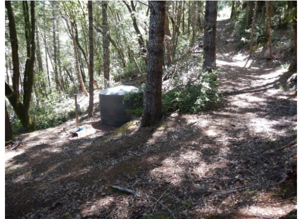
Figure 50. View of tank, onstream landing, and access road to diversion from below the house.
