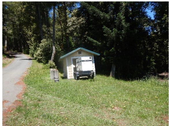
Figure 5. View of driveway and shed, with generator in front and fuel in rear.
