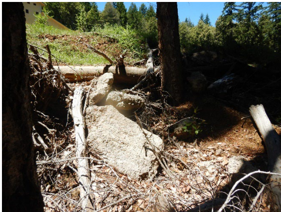
Figure 31. View of slash and logs buried by fill at outboard edge of landing, with concrete chunks.
