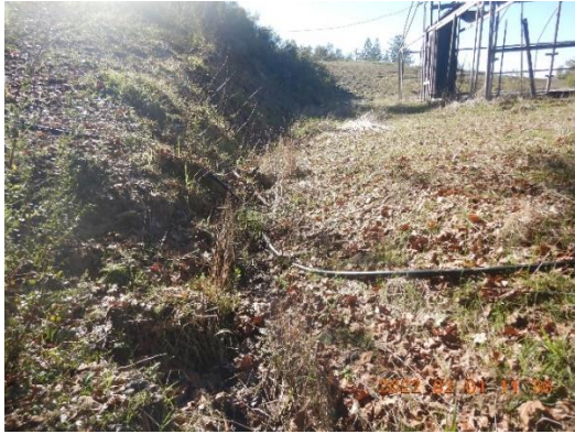
Figure 21. Picture of greenhouse, cut bank, and drainage ditch. Seep warrants a 50' setback.
