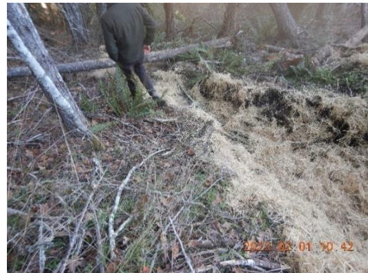
Figure 14. Outlet channel entering forested area.
