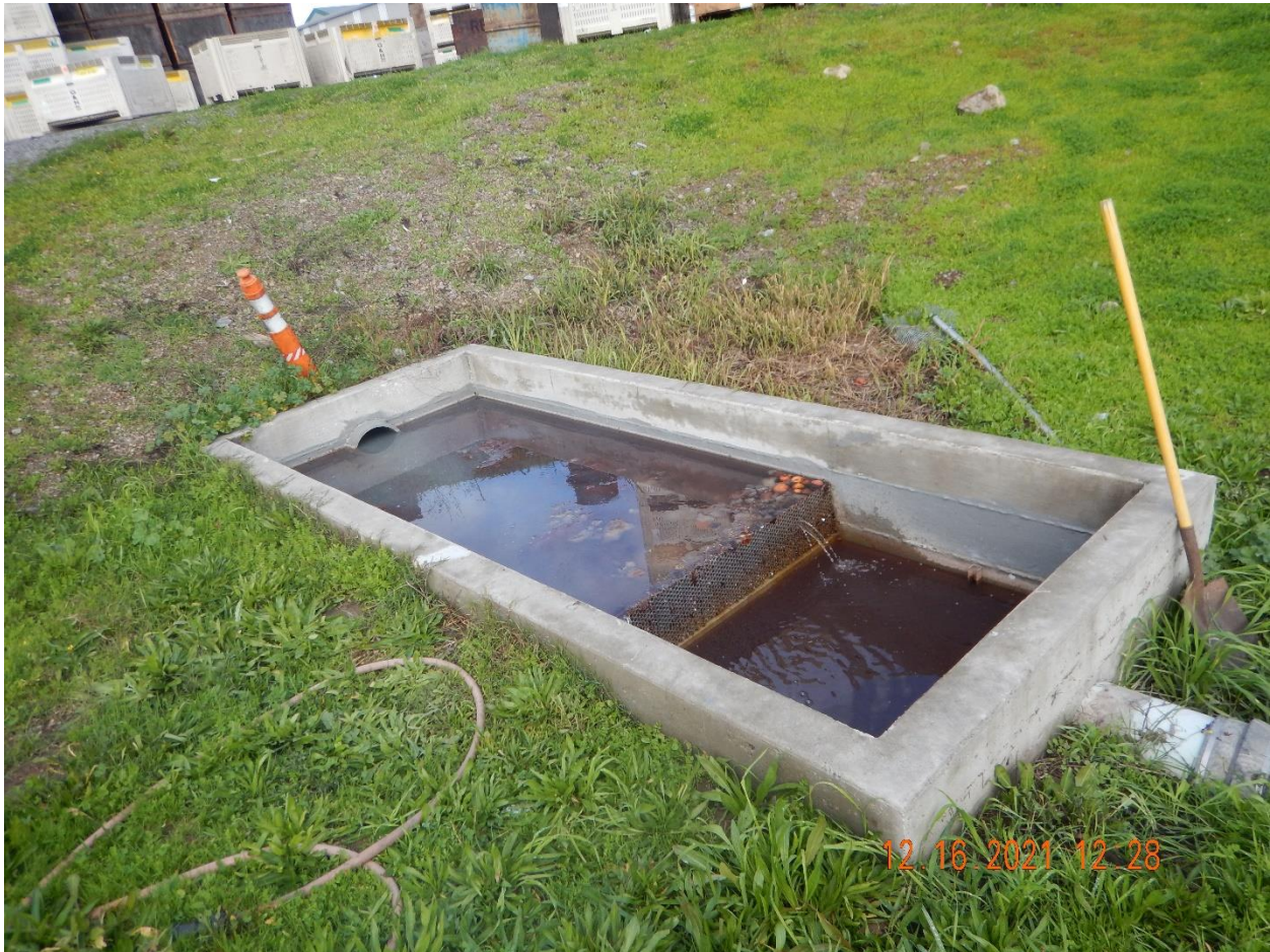
Photo 5- Concrete process wastewater sump with screen. Photo taken facing northeast.
