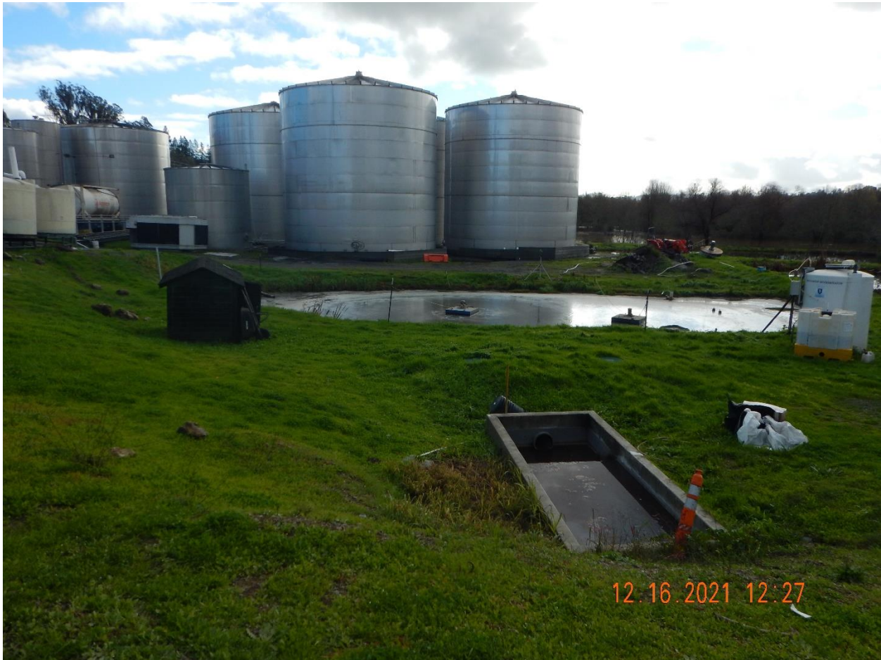
Photo 4- Process wastewater sump, septic tank risers, Pond 1 and Heritage Systems additive tank. Photo taken facing south.
