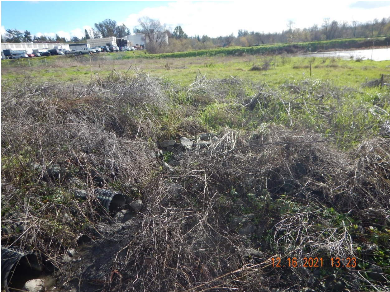
Photo 18 – Three stormwater culverts in north berm of north irrigation field, adjacent to Green Valley Road. Photo taken facing southeast.
