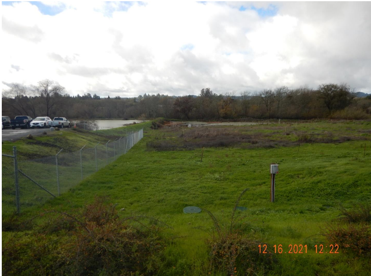
Photo 1 – Process wastewater storage pond (Pond 3), north irrigation filed, septic tank riser, mound system electric panel, and portion of mound. Photo taken facing southwest.
