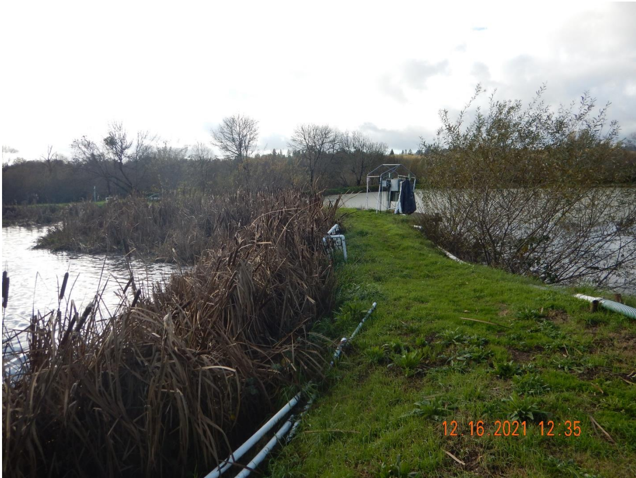
Photo 9- Berm between Pond 2 and Pond 3 with wooden platform. Photo taken facing southwest.
