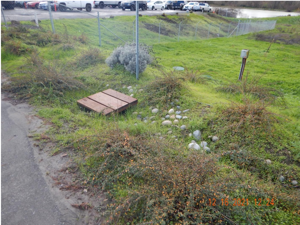
Photo 3 – Stormwater drop inlet with wood lid, at southeast corner of north irrigation field. Photo taken facing southwest.
