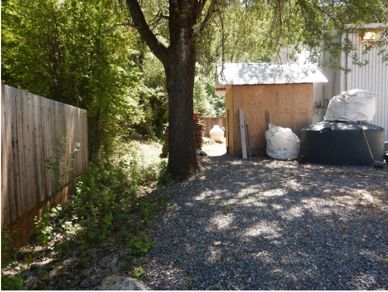
Photo 5 – Nursery/Processing Area: Side of building with propane tank, wastewater holding tank, stack of pallets, and other related equipment staged near a drainage channel.
