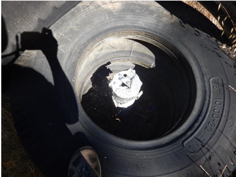
Photo 4: Well in stack of tires with duct tape partially covering top
