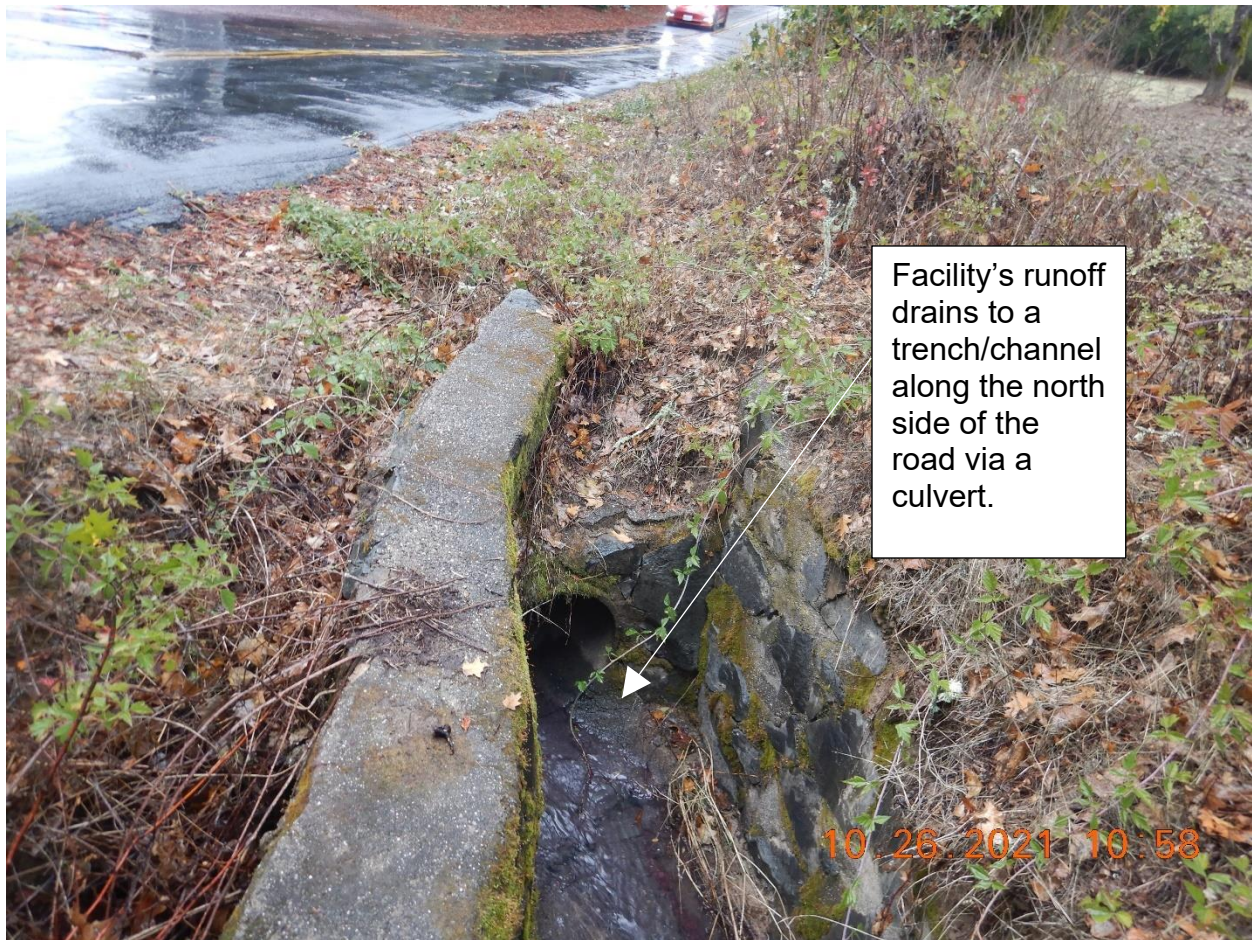
Picture 8- View of a culvert that drains the Facility's runoff into the roadside trench/channel where the samples were collected. The water appeared clear. Picture taken by Farzad Kasmaei.
