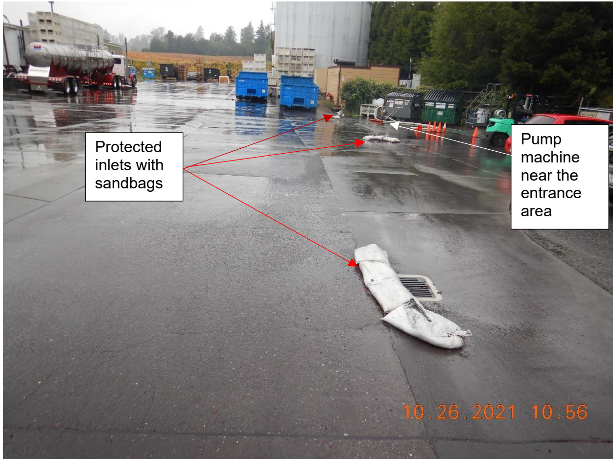
Picture 5- View of the Facility's yard and inlets protected with sandbags. Picture taken by Farzad Kasmaei.
