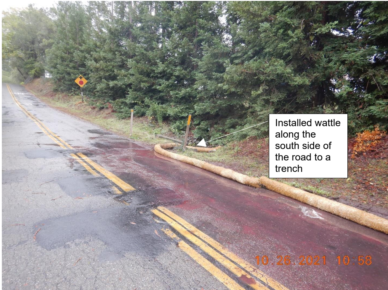
Picture 7- View of red staining in the road (Vine Hill School Road). Picture taken by Farzad Kasmaei.
