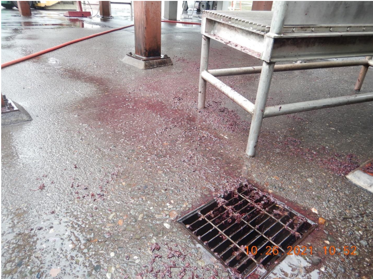
Picture 3- View of a storm drain inlet within the crush pad area. Red staining was observed on the ground. Evidence of discharged wine spill to an on-site inlet. Picture taken by Farzad Kasmaei.
