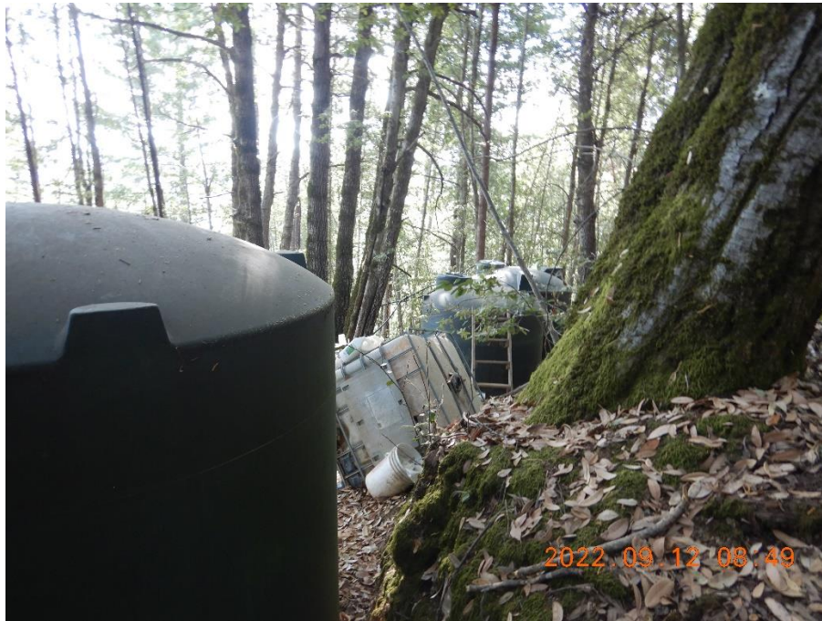
Photo 21—Water tanks located at WQ9.
