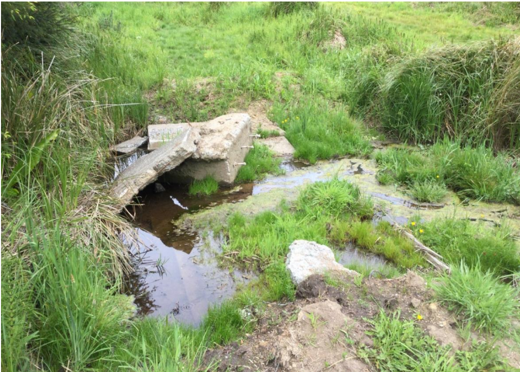
Figure 5. Unpermitted stream crossing with concrete fill. Northern red-legged frog ( Rana aurora ), a State Species of Special Concern, observed in this location.
