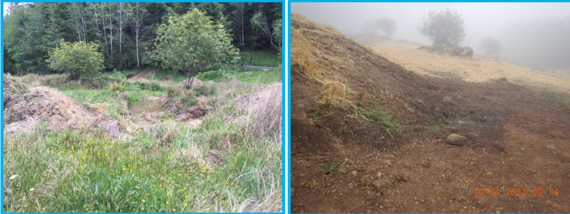
Photographs 1a and 1b. Photographs showing ongoing and increased extent of ground disturbance on northern slopes. Photograph 1a taken May 27, 2022 by Kalyn Bocast, CDFW and Photograph 1b taken during October 4, 2022 site visit by Amanda Piscitelli. Note fill adjacent to standing water and possible wetland vegetation in 1a and seep and sedges at base of jump in 1b. Both photographs taken in same general location.
