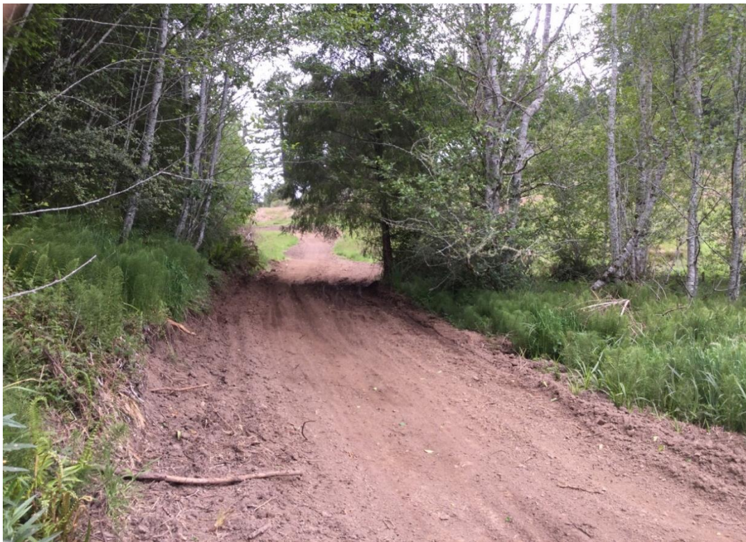
Figure 7. Grading in the headwaters of a stream/wetland complex.
