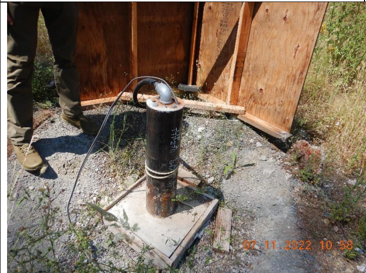
Photo 3: Ground water well at inspection point WQ3
