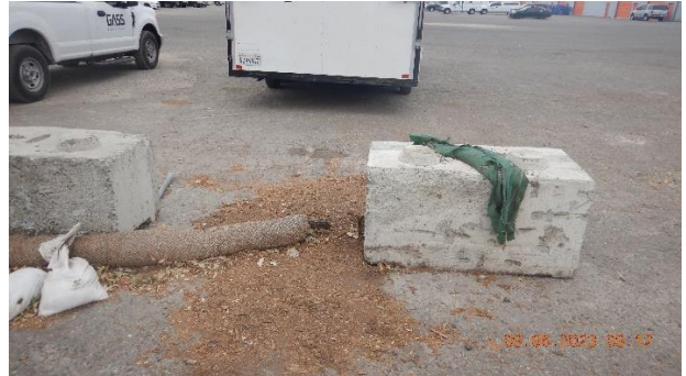
Pictures 3a, 3b - View of the wood chips on the ground showing that these fine materials can be washed off easily and discharged into the vegetated roadside ditch. Picture taken by Farzad Kasmaei.
