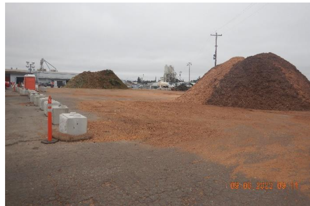
Pictures 1a, 1b - Looking north at the Facility's yard where uncovered wood chip stockpiles are stored, and wood chips was observed on the ground at the entire yard. Both pictures indicate an ineffective perimeter control BMP installation. Picture taken by Farzad Kasmaei.
