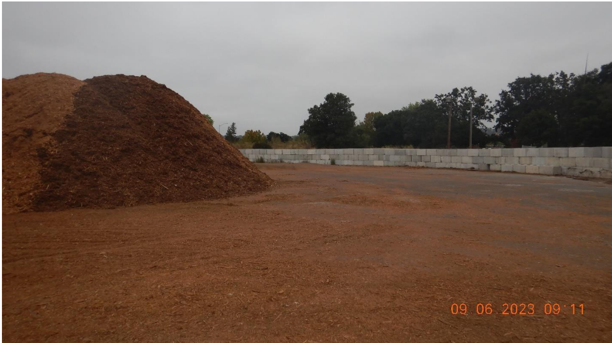
Picture 2- View of significant amount of wood chips on the paved area. Picture taken by Farzad Kasmaei.
