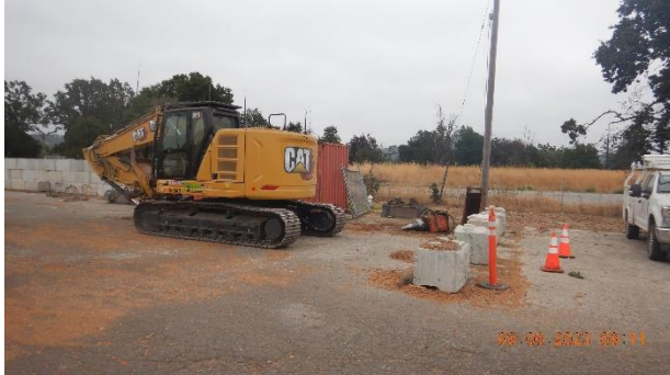
Pictures 3a, 3b - View of the wood chips on the ground showing that these fine materials can be washed off easily and discharged into the vegetated roadside ditch. Picture taken by Farzad Kasmaei.
