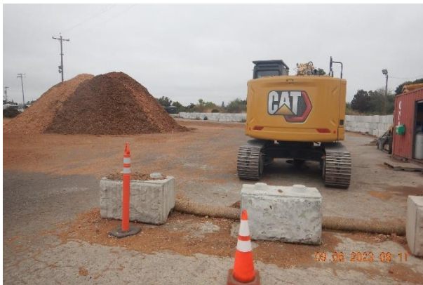
Pictures 1a, 1b - Looking north at the Facility's yard where uncovered wood chip stockpiles are stored, and wood chips was observed on the ground at the entire yard. Both pictures indicate an ineffective perimeter control BMP installation. Picture taken by Farzad Kasmaei.
