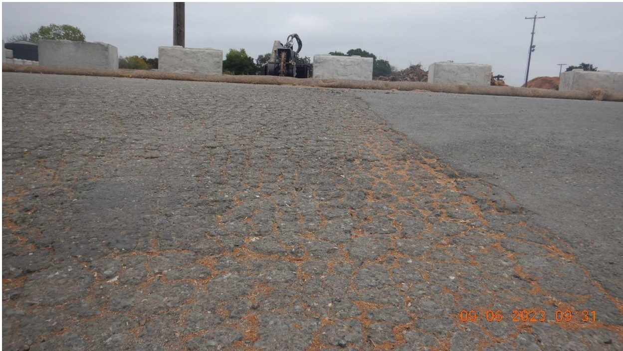
Picture 9 – View of the paved area off-site that indicates wood chips mobilization due to the BMP deficiencies. Picture taken by Farzad Kasmaei.
