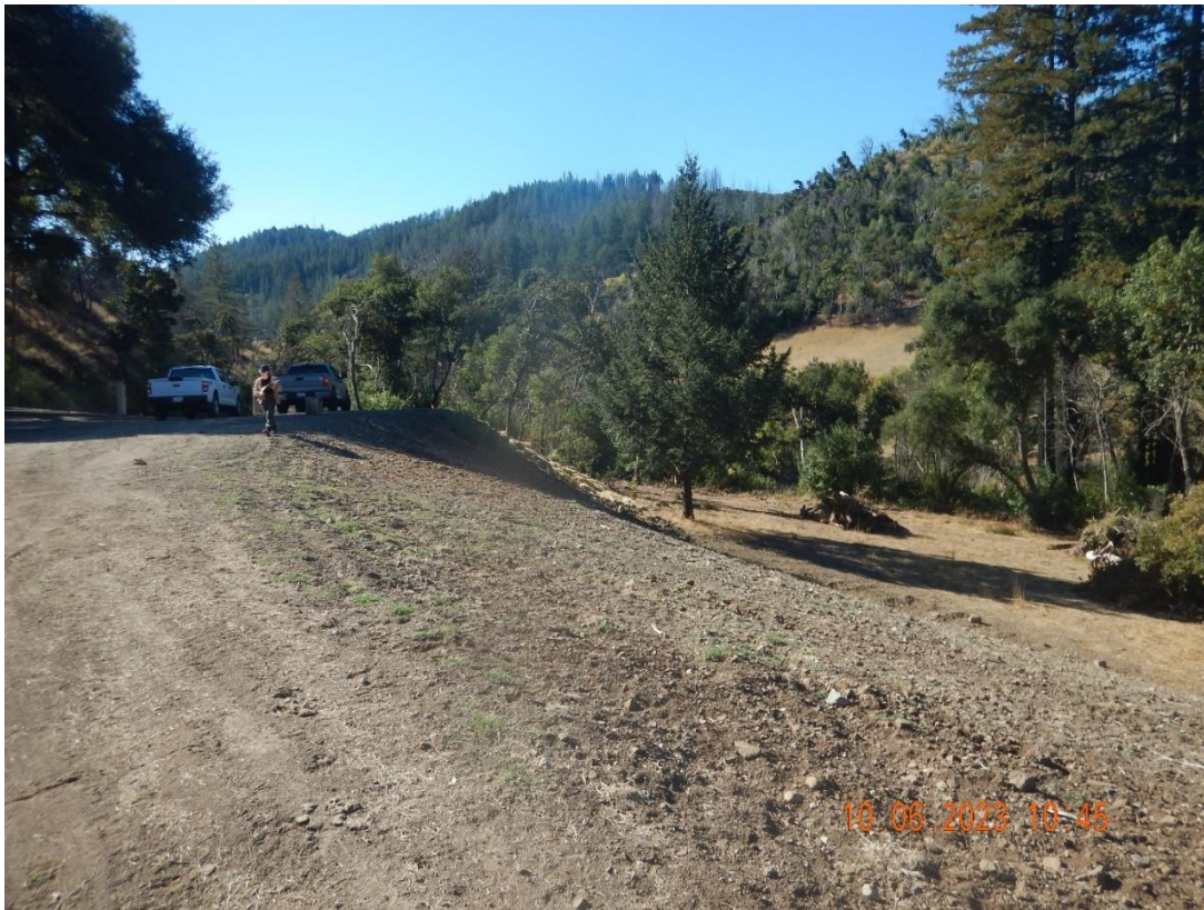
Photo 2: Fill area, looking south with Mark West Creek to the right.
