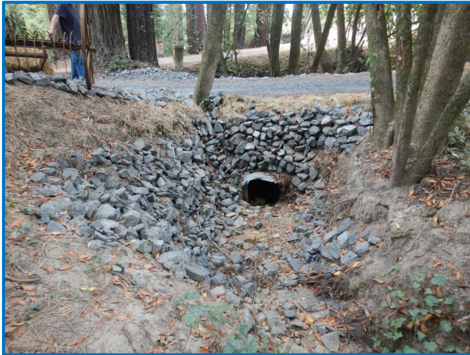
Photograph 2: Photograph of complaint site's streambanks, road fill face and culvert inlet. Some rock used to stabilize steep banks that has failed into the stream.
