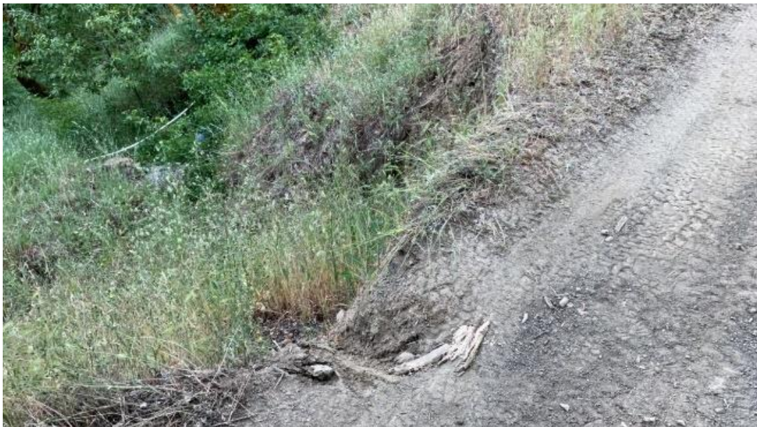
Figure 49. outlet of X4 crossing (facing E).
