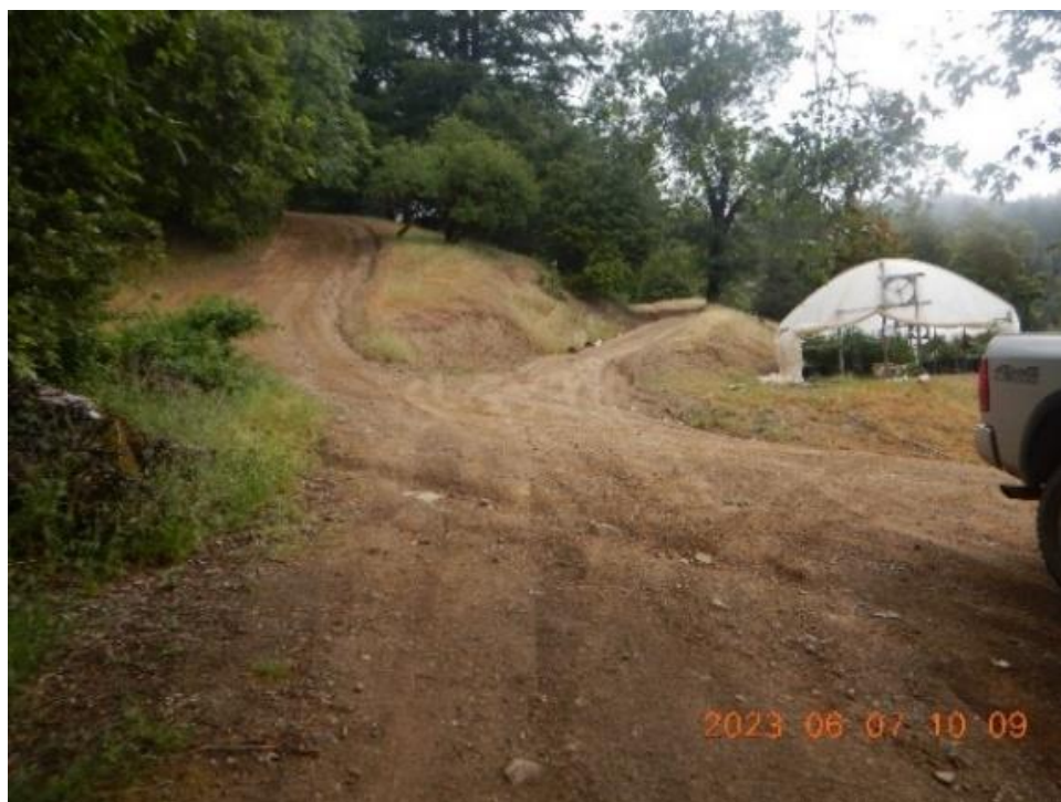
Figure 7. X1. Road sediment delivery from two upslope road segments. CA1 is cultivation area near X1.
