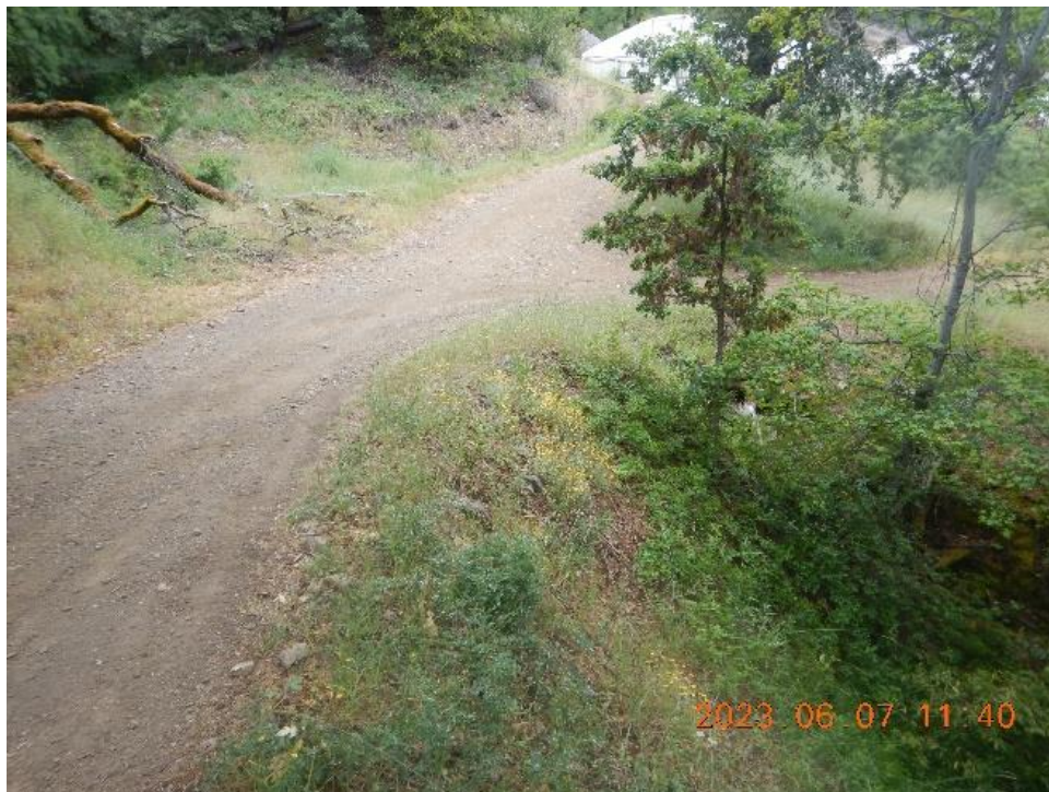
Figure 32. Road over stream crossing X3.
