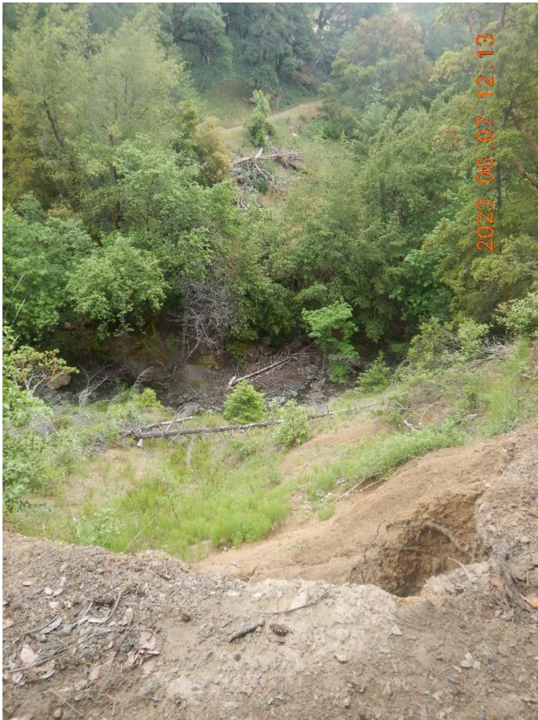
Figure 21, Road related slide delivery to the blue line watercourse.
