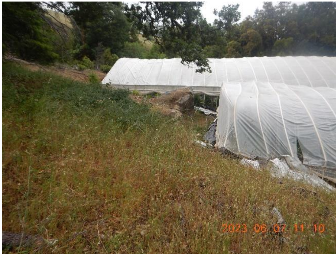
Figure 37. Upslope of CA3, the cut bank appears to have failed.
