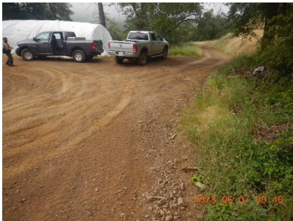
Figure 8. Road runoff flows past greenhouses and delivers to the watercourse downslope of the crossing at X1.
