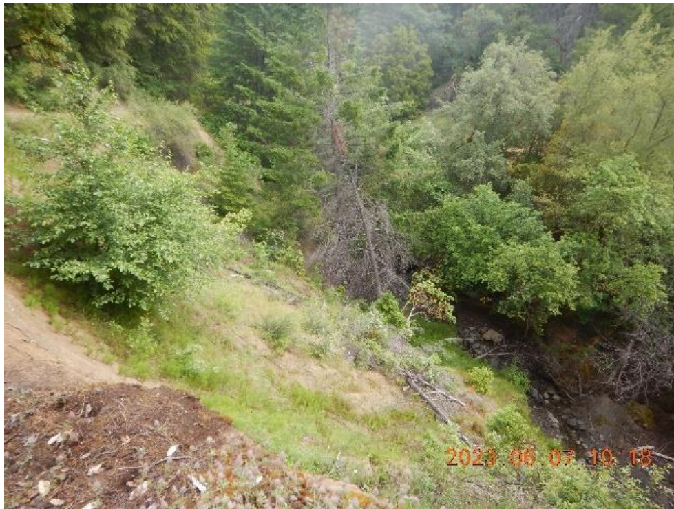
Figure 22. Unstable slope leading directly to watercourse.
