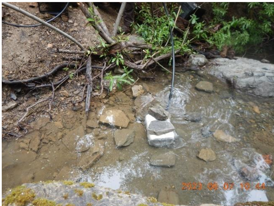
Figure 29. Diversion line at X2 culvert outlet.
