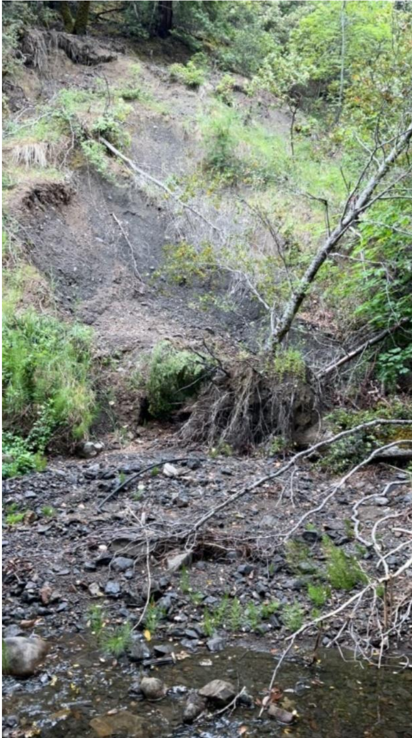
Figure 26. Slide located on the right bank upstream of X2 inlet.
