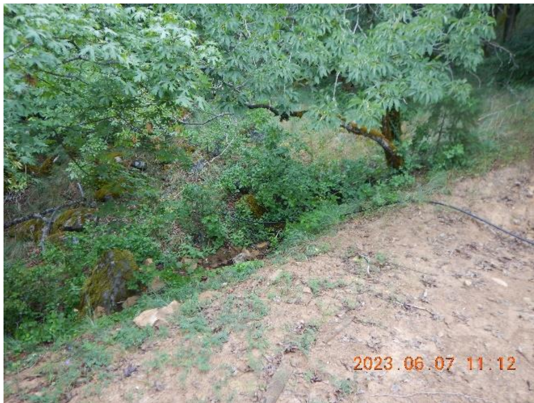
Figure 41. Graded area on Class II watercourse.
