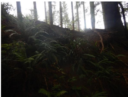
Figure 13. View from watercourse of left bank with fill pushed to the top of the bank and riparian forest removed.
