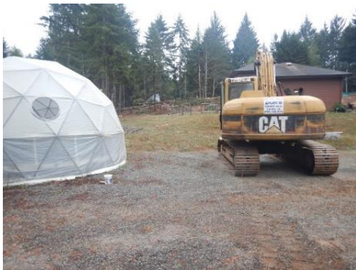
Figure 45. Excavator onsite rented from Don's Rent All.
