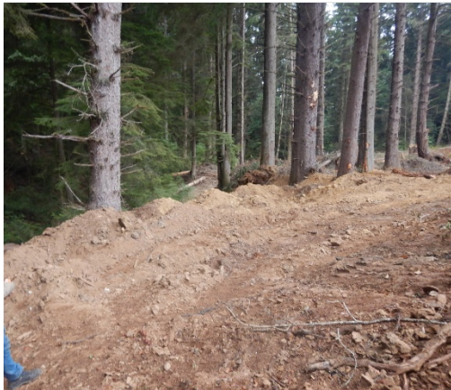
Figure 33. Fill placed in riparian area near WP960.
