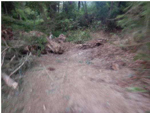
Figure 22. At WP958, the road arrives at the watercourse where stumps and root wads were placed in the watercourse.
