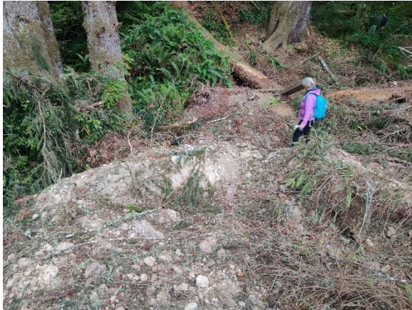
Figure 11. Fill pushed onto left bank of watercourse near WP 949. Photo by Jesse Cahill on September 27, 2022.
