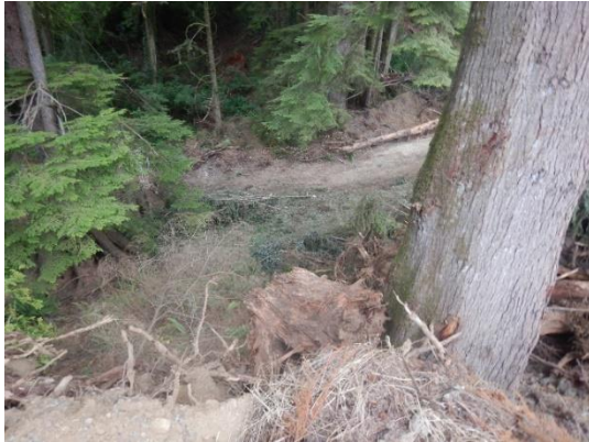
Figure 38. View down at road between WP957 and WP958.
