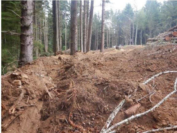
Figure 32. Fill placed in riparian area near WP960.
