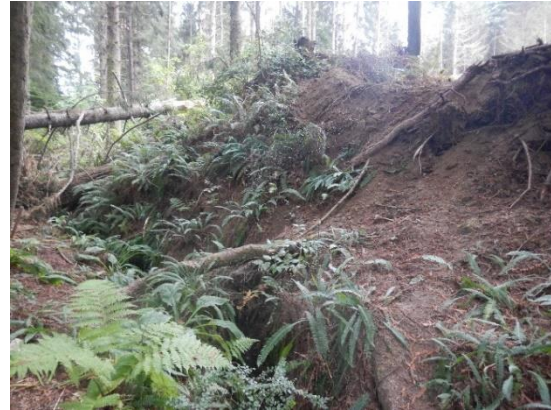
Figure 14. Fill placed on left bank above channel near WP956, over a 25' channel length.
