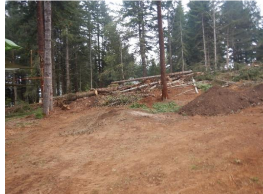
Figure 47. View toward southern Property boundary with harvested trees and piled fill.
